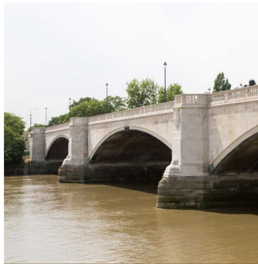
Restoration of Chiswick Bridge is complete
