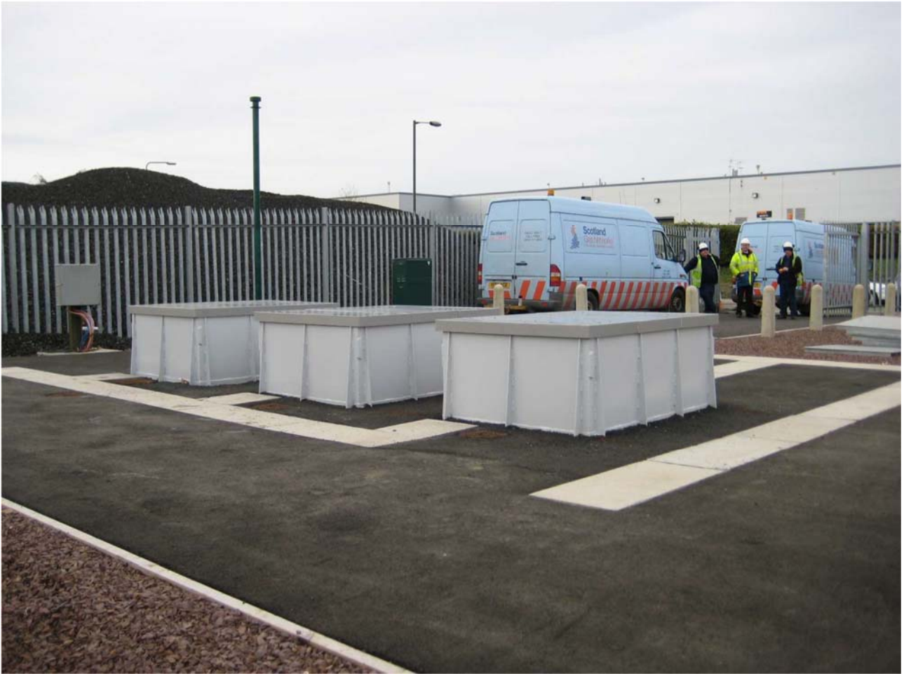
Figure 3 – Illustrative photograph of a standard SGN Gas PRS, of the type to be installed (note that the PRS proposed for Greenwich involves only two of the grey cabinets rather than the three in the image)
