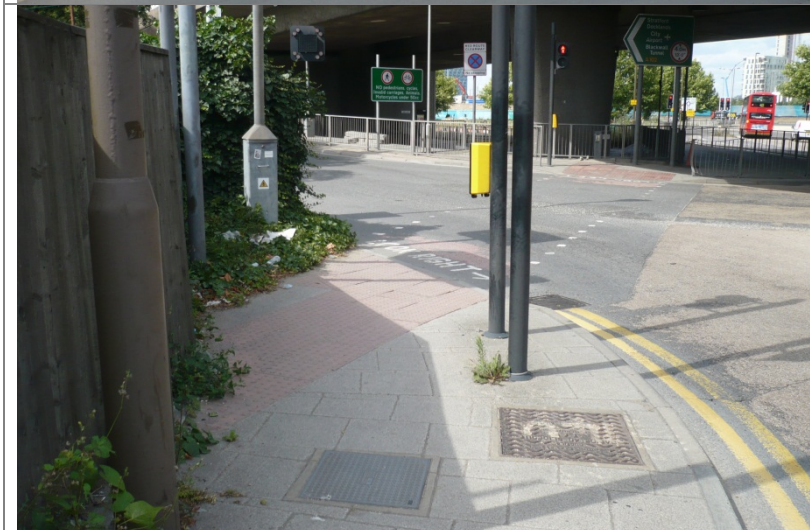
Crossing 9 (Blackwall Lane slip road): very narrow approach to the crossing, overgrown vegetation, fast moving traffic, limited waiting areas, rutted tarmac (tripping hazard)
