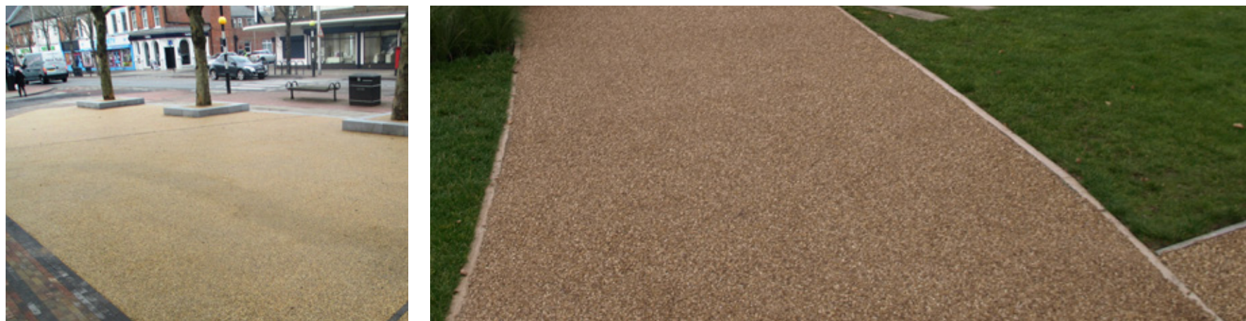
Figure 5.13. Paving materials may include resin bound gravels which are low maintenance but high quality.
