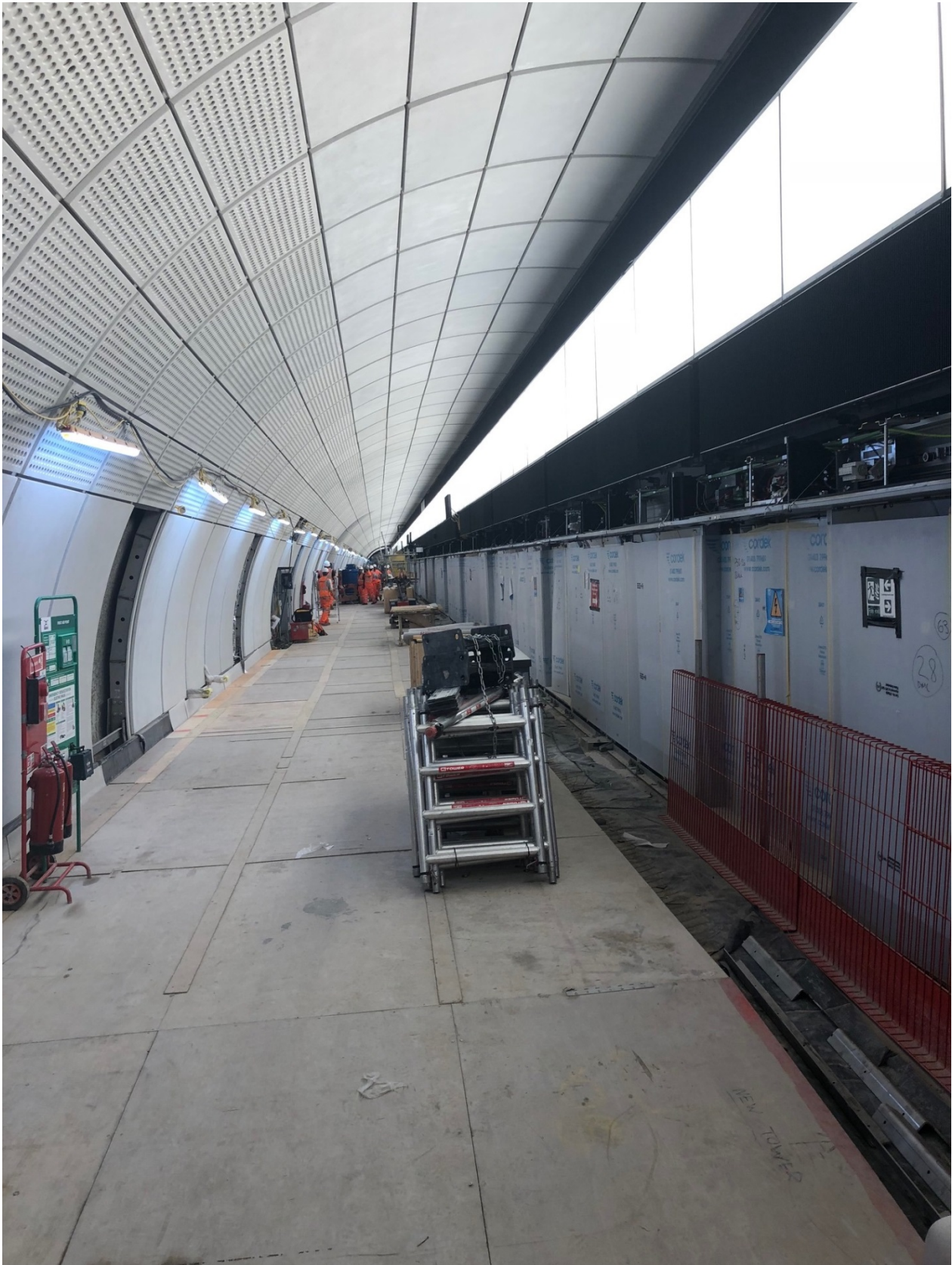
Whitechapel station platform (installation of platform edge screens)
