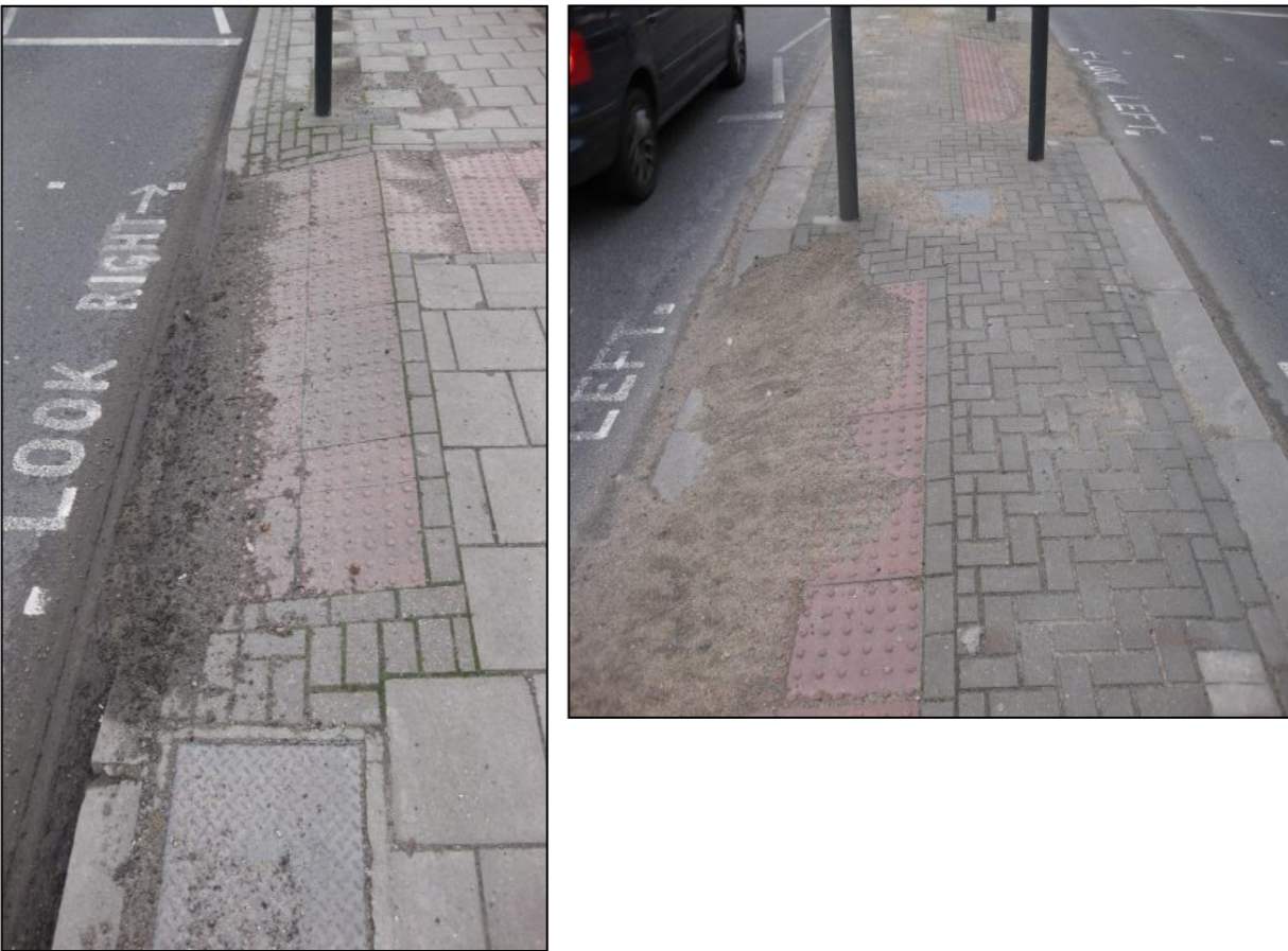
FIGURE 3.26 PHOTOGRAPHS OF CROSSING 5-A
