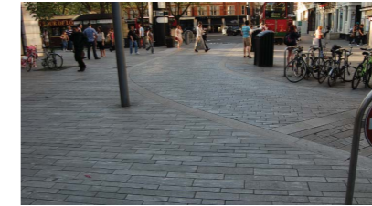
1. Raised and paved carriage way (Granite setts)
