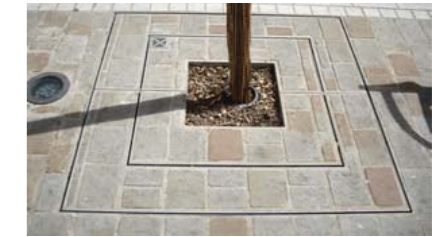
6. Wide kerb around the grassed area
