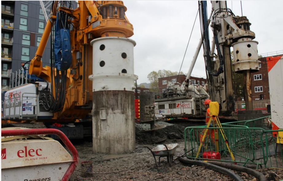
Piling in progress
