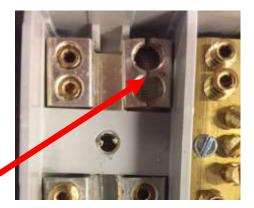
'Splitting' in the phase terminal block
