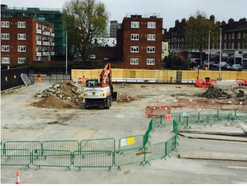
5) Tarmac removal and piling mat excavation
