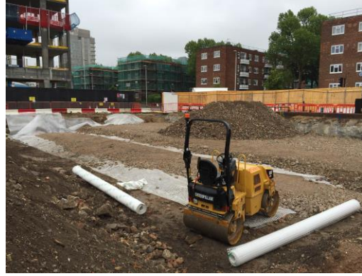
6) Piling mat construction
