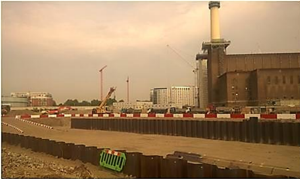
Battersea Crossover Box sheet piling operation completed
