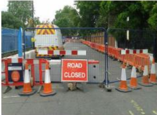
3) Closing of Road for Gas Diversion
