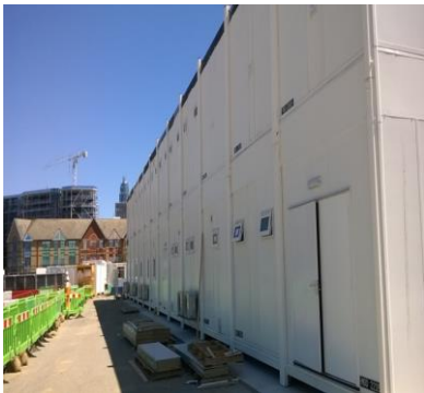
Site Accommodation Establishment
