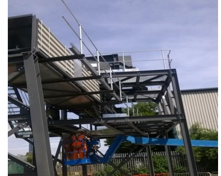
Conveyor Belt installation
