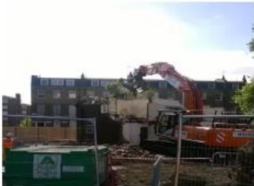
2) Demolition of Lodge
