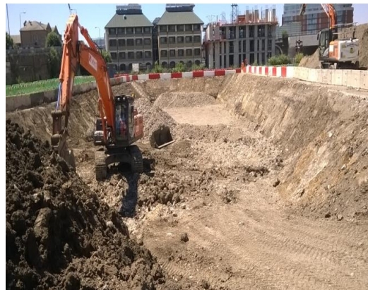
Removal of obstructions within Station Box left behind from previous industrial use
