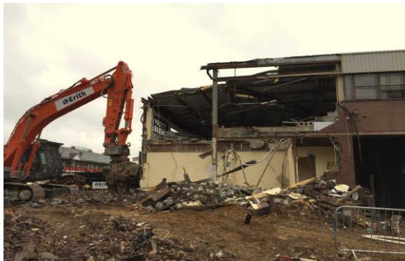
9) Covent House demolition
