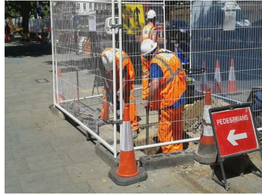
5) Service trial holes
