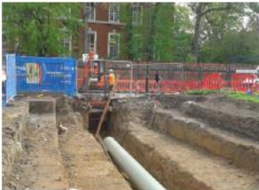
4) Laying New Gas main
