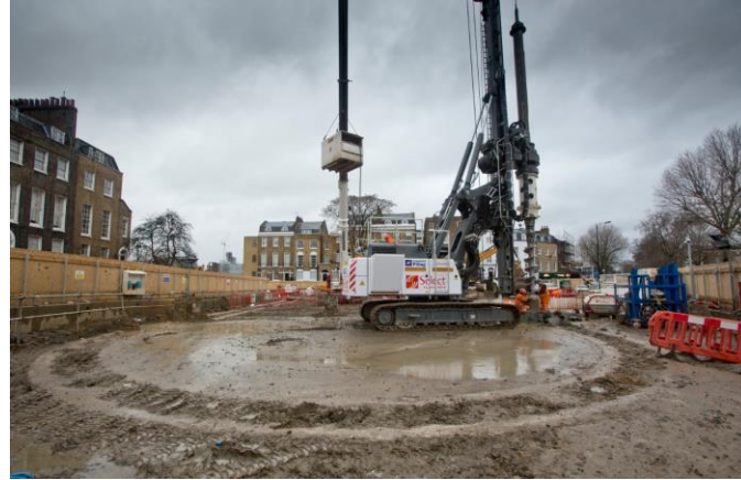
KG shaft overview
