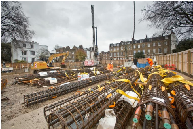
Overview of cast material for piling
