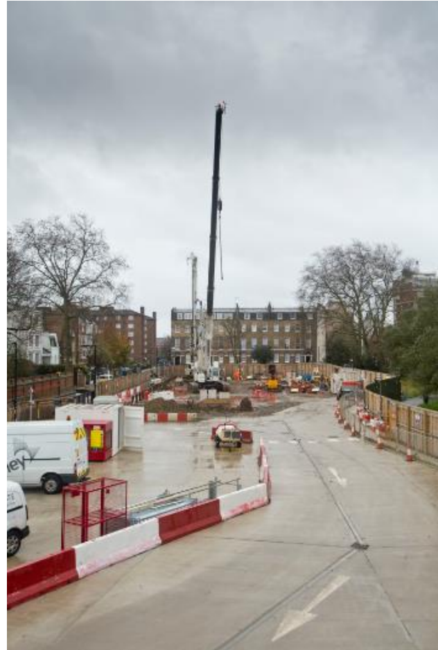
Piling operating at Kennington Park site
