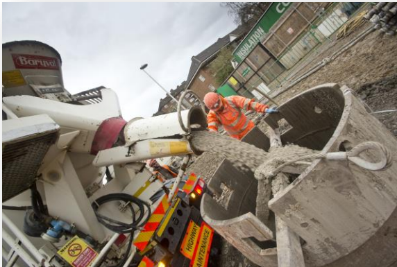
Concrete activity ongoing at Nine Elms
