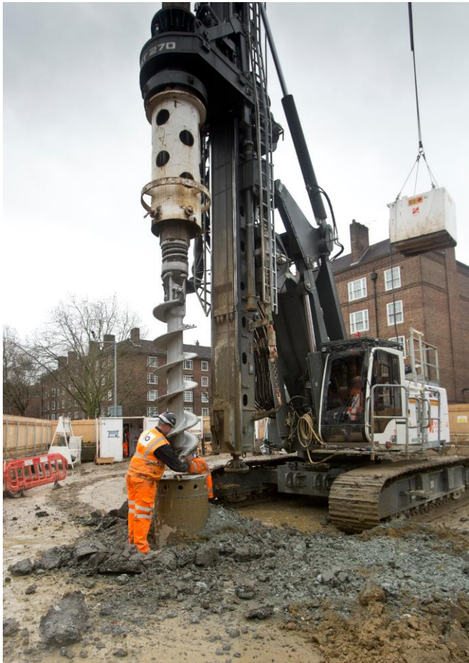
FLO technical operating piling rig
