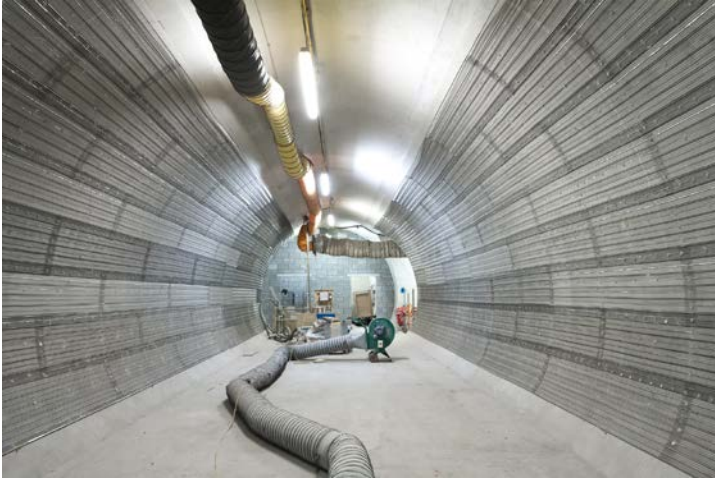
Tottenham Court Road station's Central line interchange tunnel
