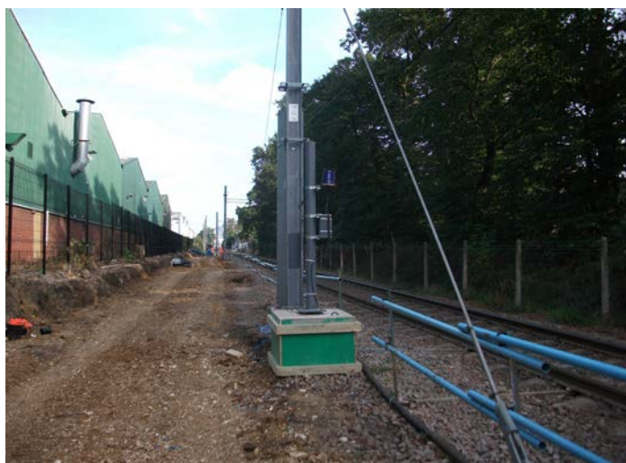
Twin tracking works
