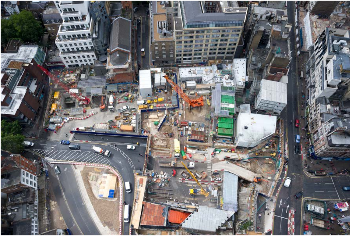
Aerial view of the Tottenham Court Road site
