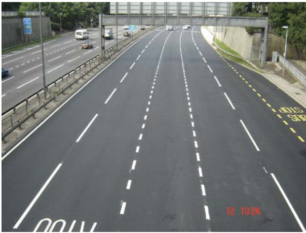
A406 five lanes Eastbound at High Road Bridge
