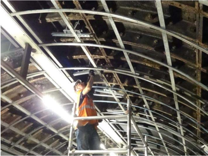
Unistrut bracket installation at Vauxhall station
