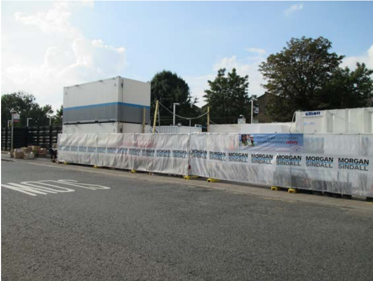
Kensal Rise station site set up
