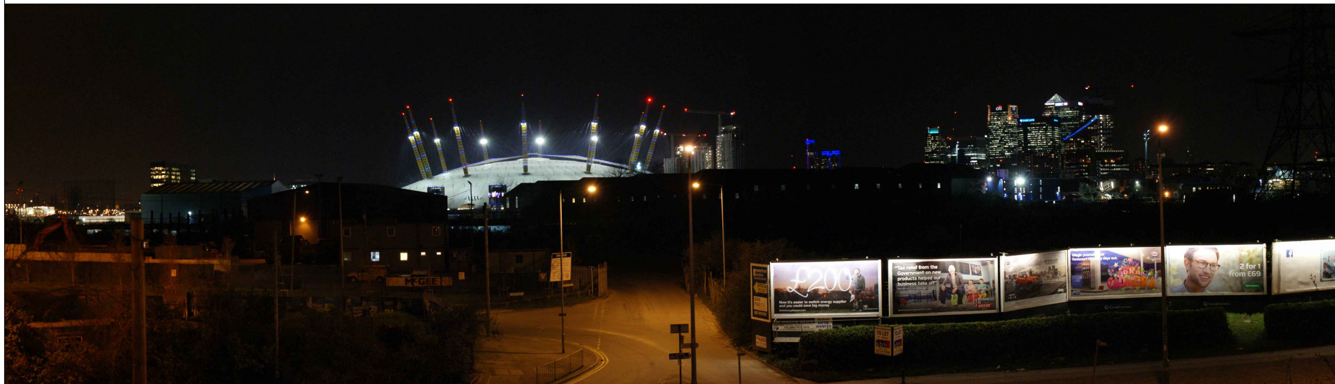
VIEWPOINT 1 - NIGHT TIME VIEW FROM SILVERTOWN WAY AT JUNCTION WITH LOWER LEA CROSSING, LOOKING SOUTH WEST
