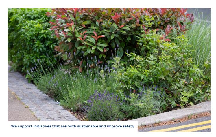
in our Climate Change Adaptation Plan. The new drainage system measures at these locations include a green roof, rain gardens and permeable paving and will help to reduce surface water flood risk, as well as support biodiversity.
