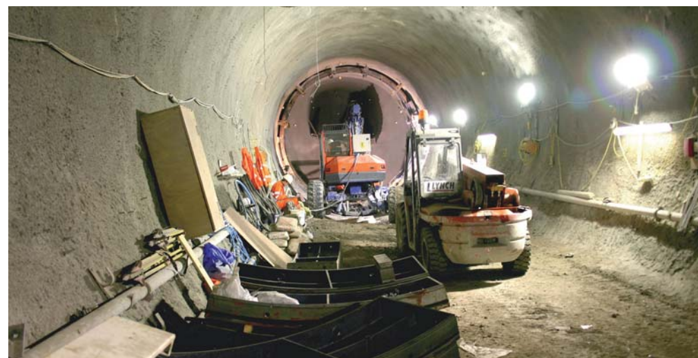
Piccadilly line tunnelling
