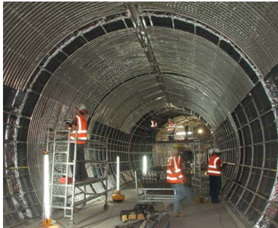
Underground passenger tunnels under construction © Balfour Beatty Civil Engineering Ltd
