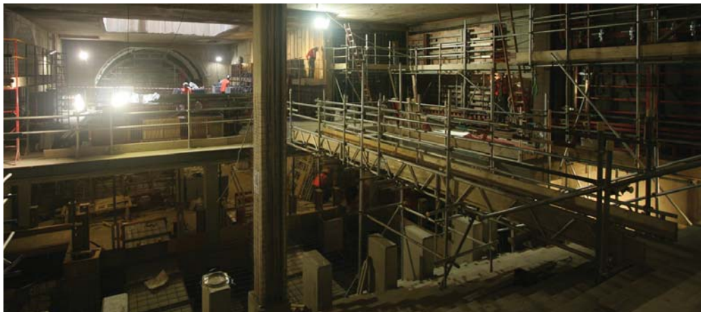
Northern ticket hall (under construction) © Balfour Beatty Civil Engineering Ltd
