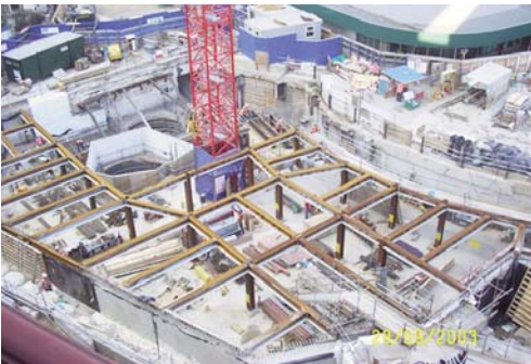
Tube ticket hall Construction image
