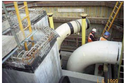
WTH – Gas main diversion
