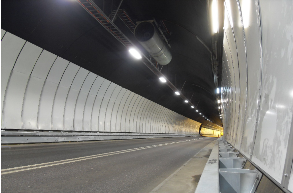
Figure 2.2: Cuilfail Tunnel in Lewes
