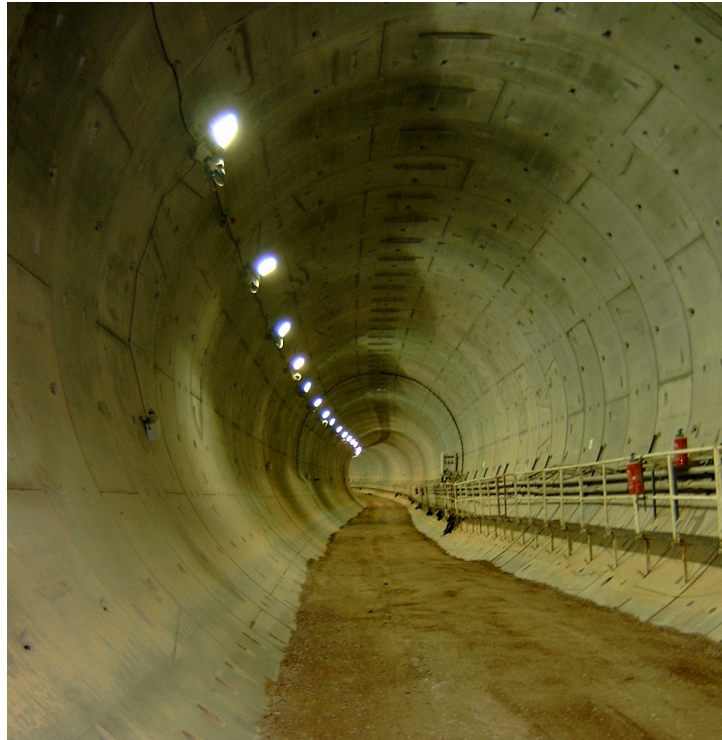
Figure 2.1: Airside Road Tunnel at Heathrow Airport
