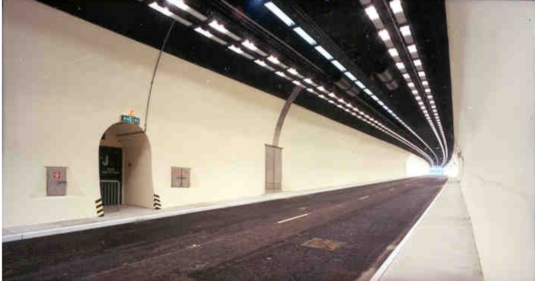
Figure 2.3: Round Hill Tunnel on the A20
