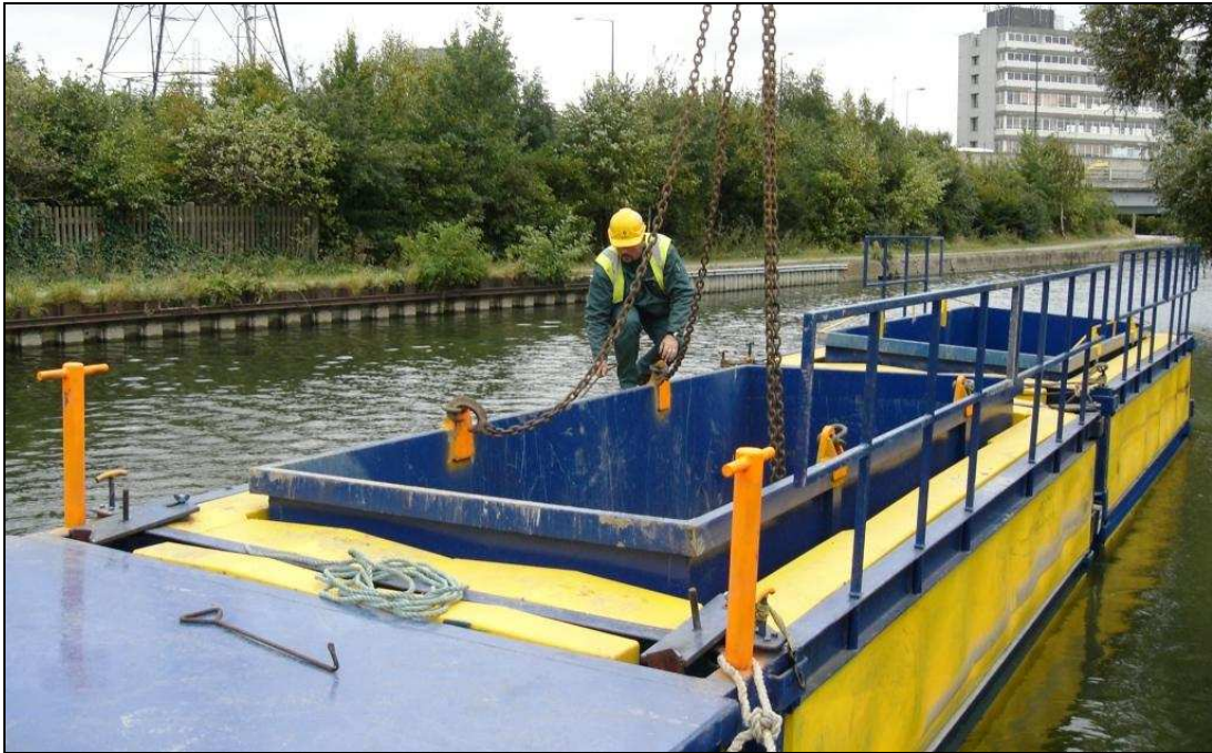
Figure 4: Smart Barge units having skips unloaded
