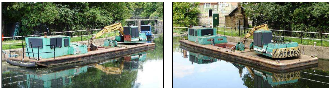
Figure 17: Barge mounted excavator crane
