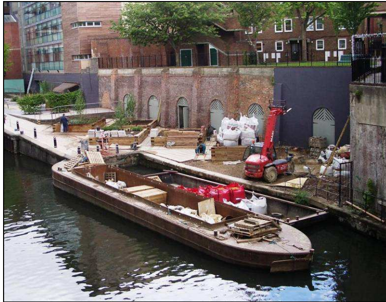
Figure 22: Forklift hoist used to unload/load barges
