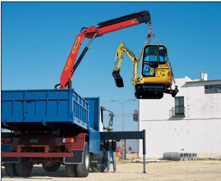
Figure 16: Example of lorry mounted telescopic crane working
