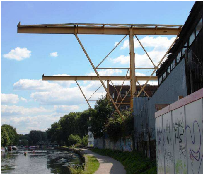
Gantry type cranes located on Watermint Quay
