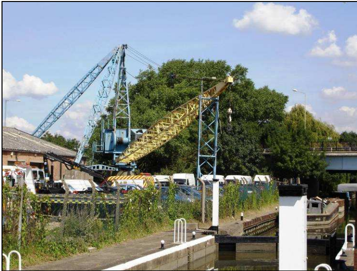
Figure 14: Examples of disused fixed cranes on the Lee Navigation
