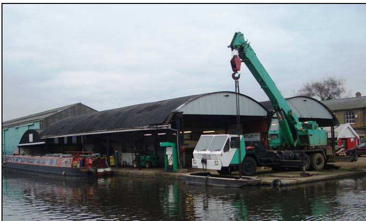
Figure 10: Wheeled crane used for lifting canal boats at a GUC boatyard
