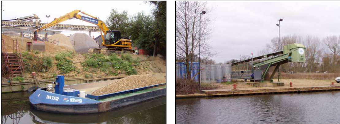
Crawler excavator with clam shell bucket Conveyor and pouring hopper
