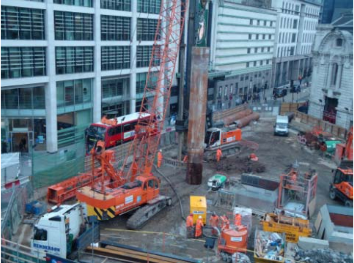
Victoria South Ticket Hall piling works
