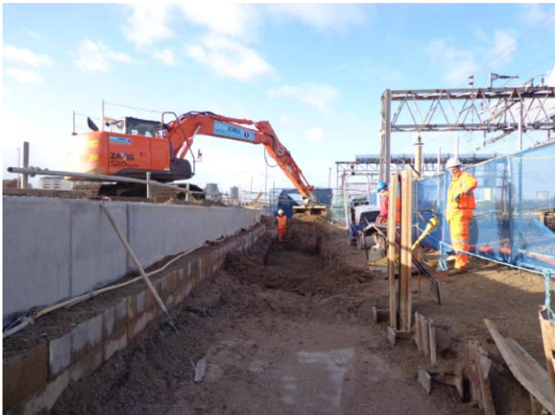
Twin tracking infrastructure works
