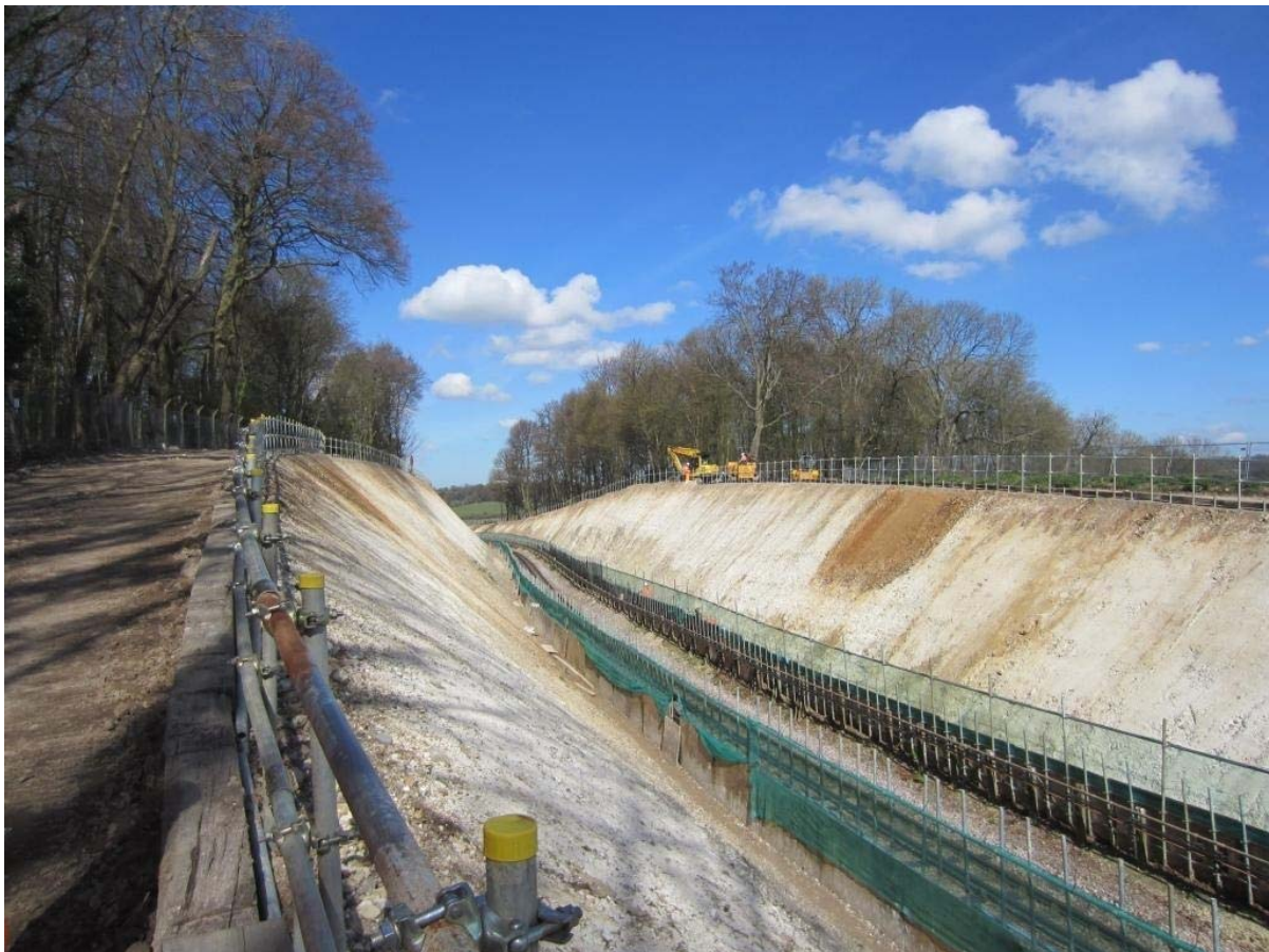
Cutting stabilisation works in progress between Chalfont and Latimer and Chesham
