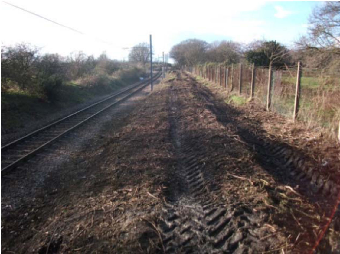
Vegetation clearance between Beddington Lane and Mitcham Junction
