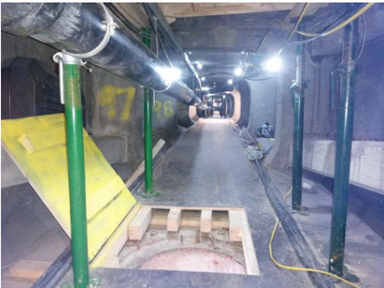
Inside Hammersmith Flyover
