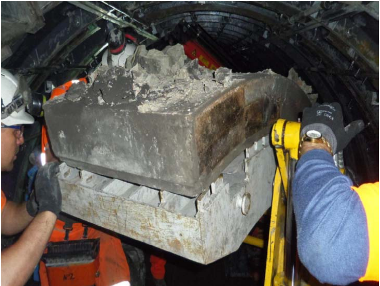
Shoulder tunnel segment on cradle
