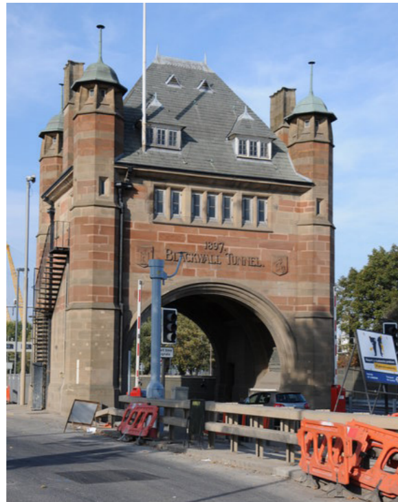
Figure 2.15 The Blackwall Tunnel Gatehouse and Millennium Square
