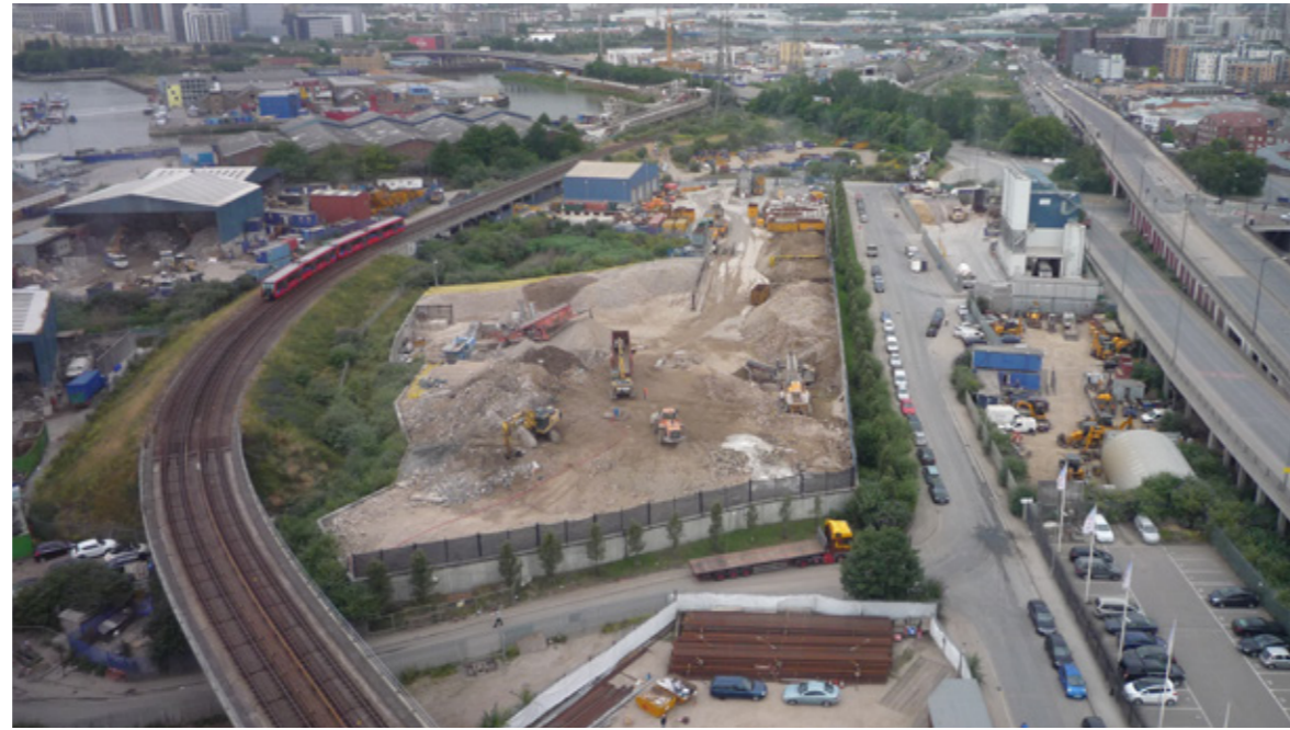
Figure 2.12 Silvertown (Northern) portal - current urban context as viewed from the Emirates Air Line and the Siemens Crystal
