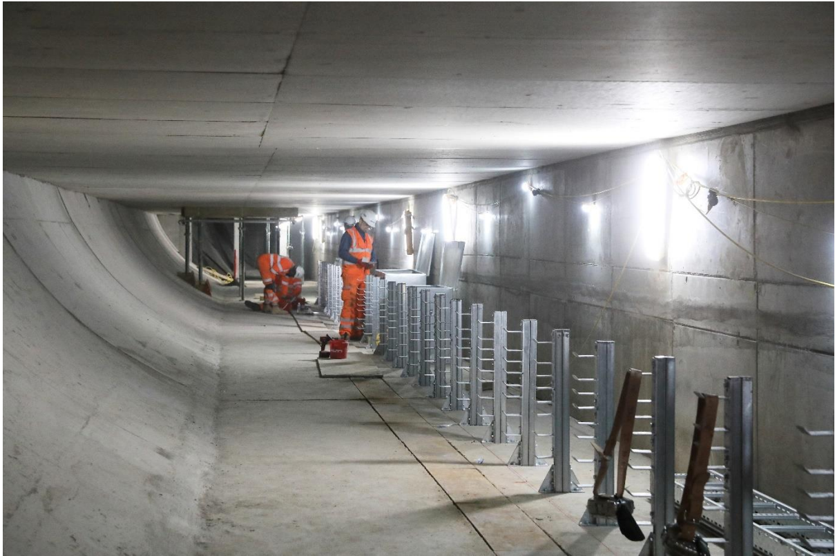
Figure 3: Installation of services below new platform
