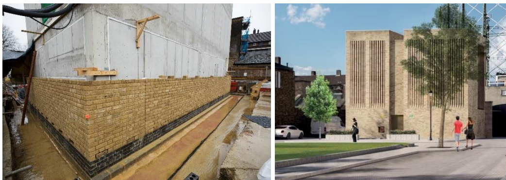
Figs 7 & 8- Progress of the Kennington Green headhouse cladding, and an artist's impression of the same at completion.
