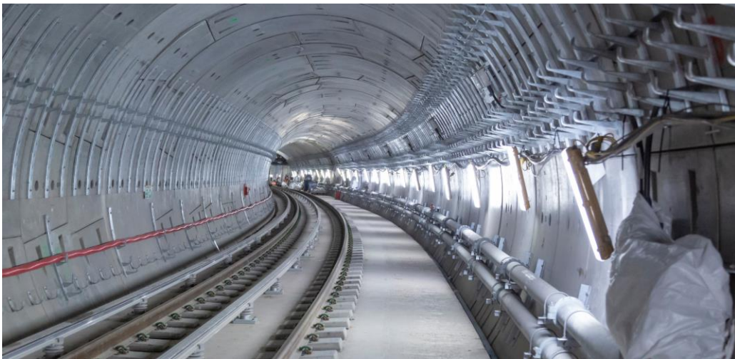
Fig 1: The southbound NLE running tunnel, with track installation completed
