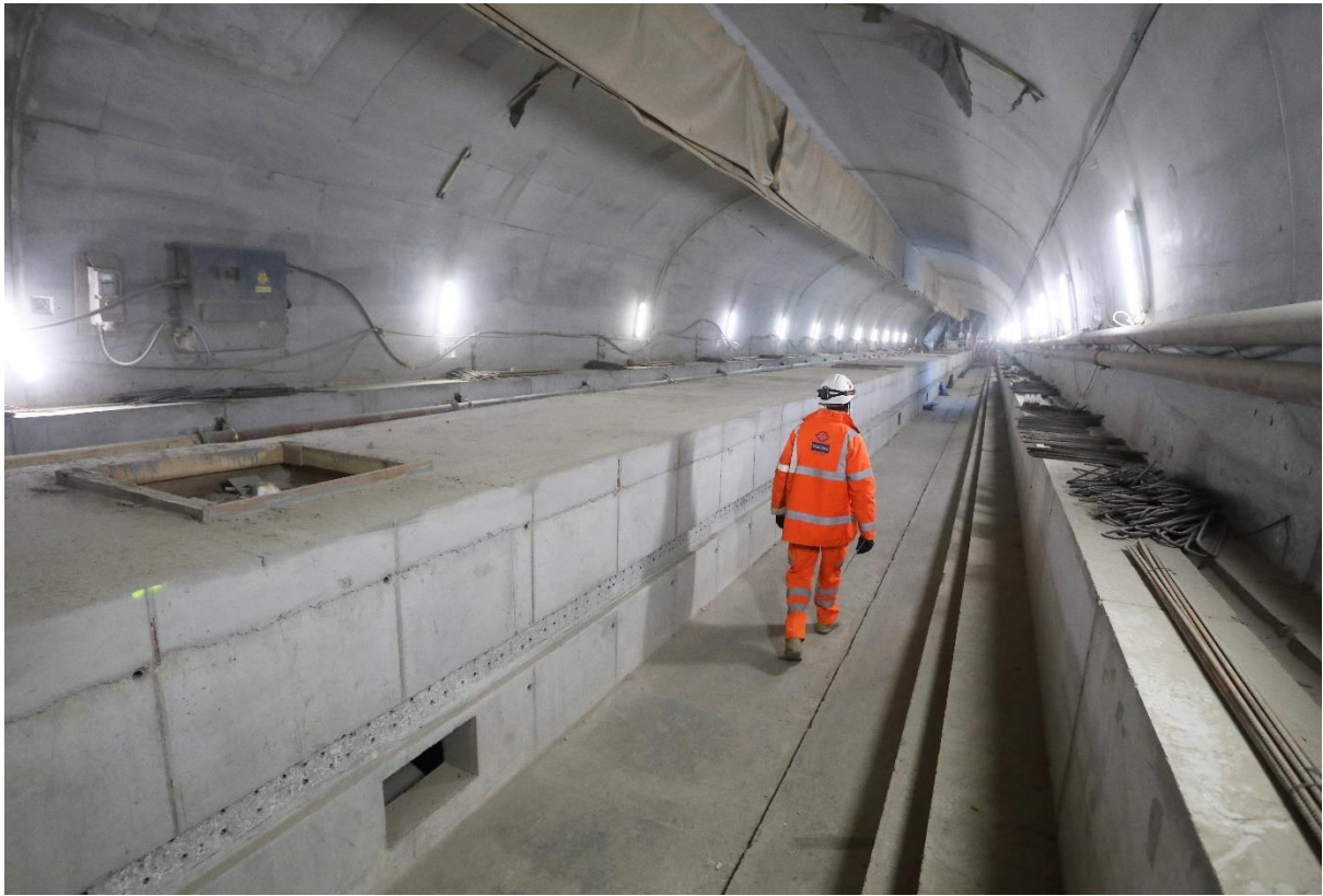
Figure 1: Moving walkway Central line-Northern line interchange link
