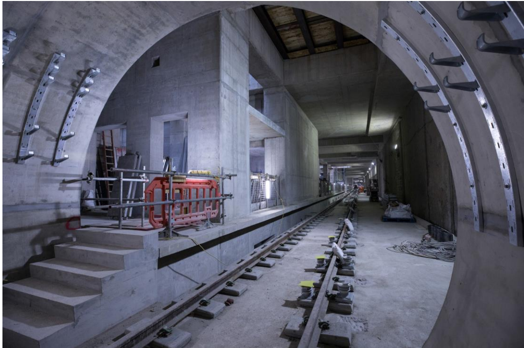
Fig. 6: An equipment room under construction at Nine Elms station.
