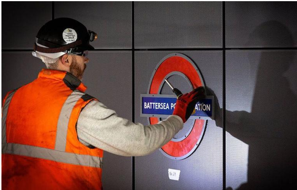
Fig. 2: A contractor installs signage at Battersea Power Station.
