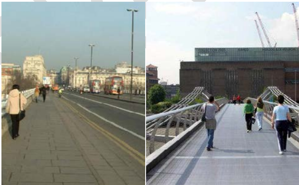
Figure 23 – Waterloo Bridge and pedestrian bridge (Millennium)
