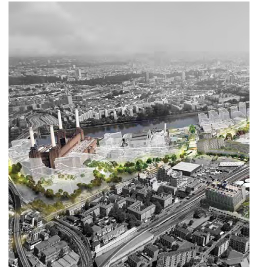
Transport investment unlocks growth areas, such as the proposed scheme for Battersea and Nine Elms
