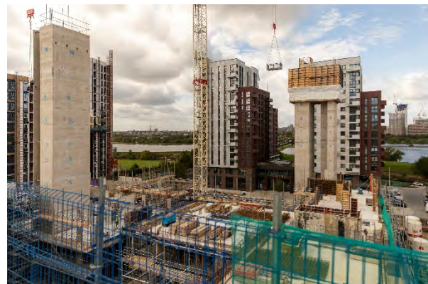
Figure 29: Blackhorse Road car park development - pre and during construction
