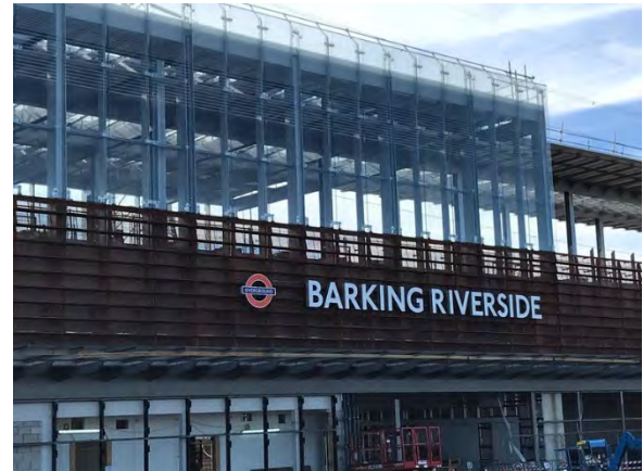
Figure 27: Barking Riverside station entrance
