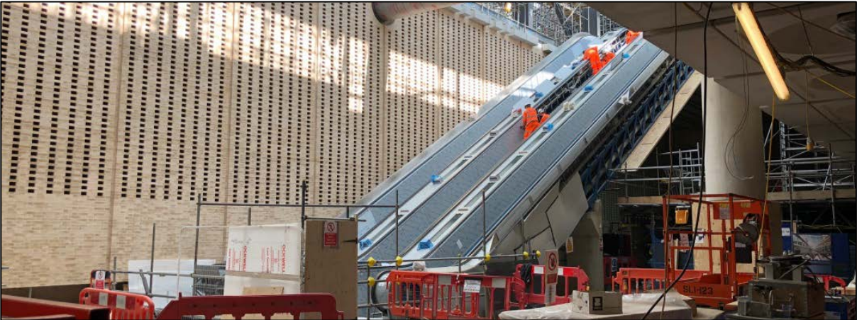
Installation of Escalators at Paddington Station
