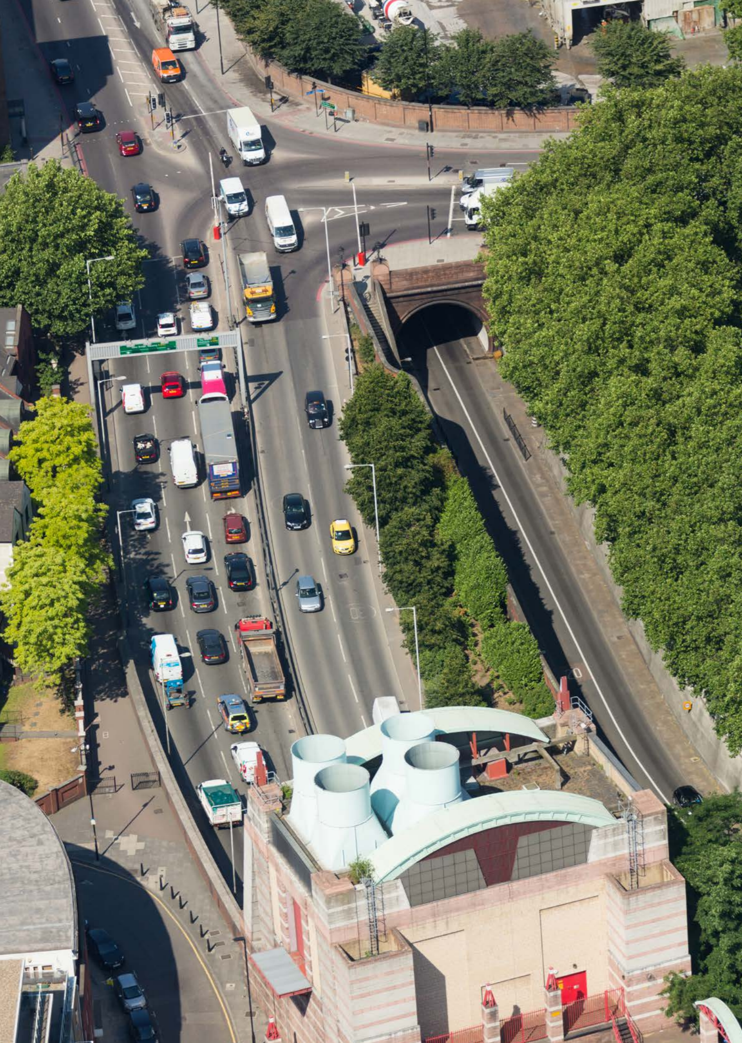
The design of the refurbished Rotherhithe Tunnel is complete
