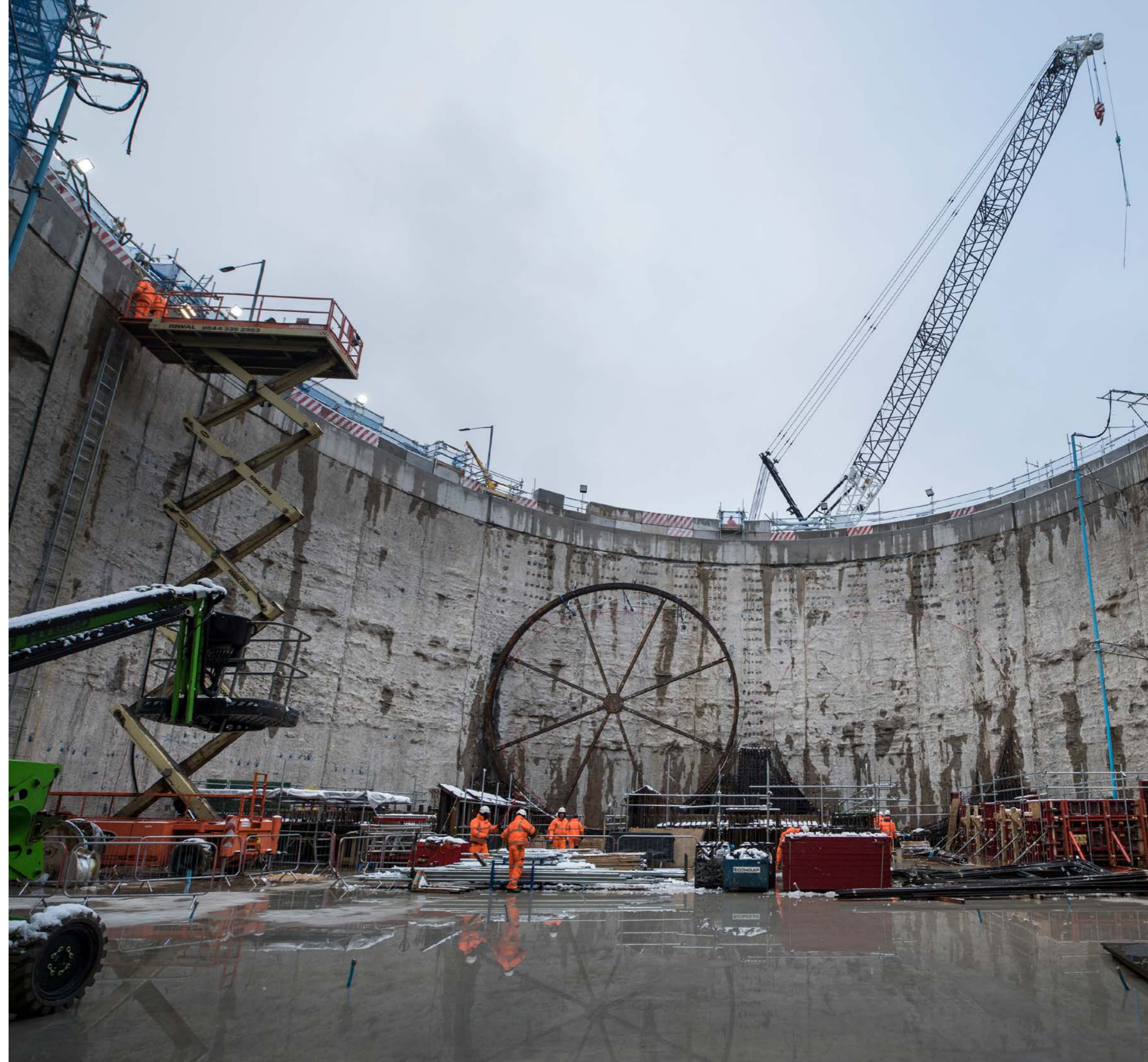
We're working on the southbound section of the Silvertown Tunnel
