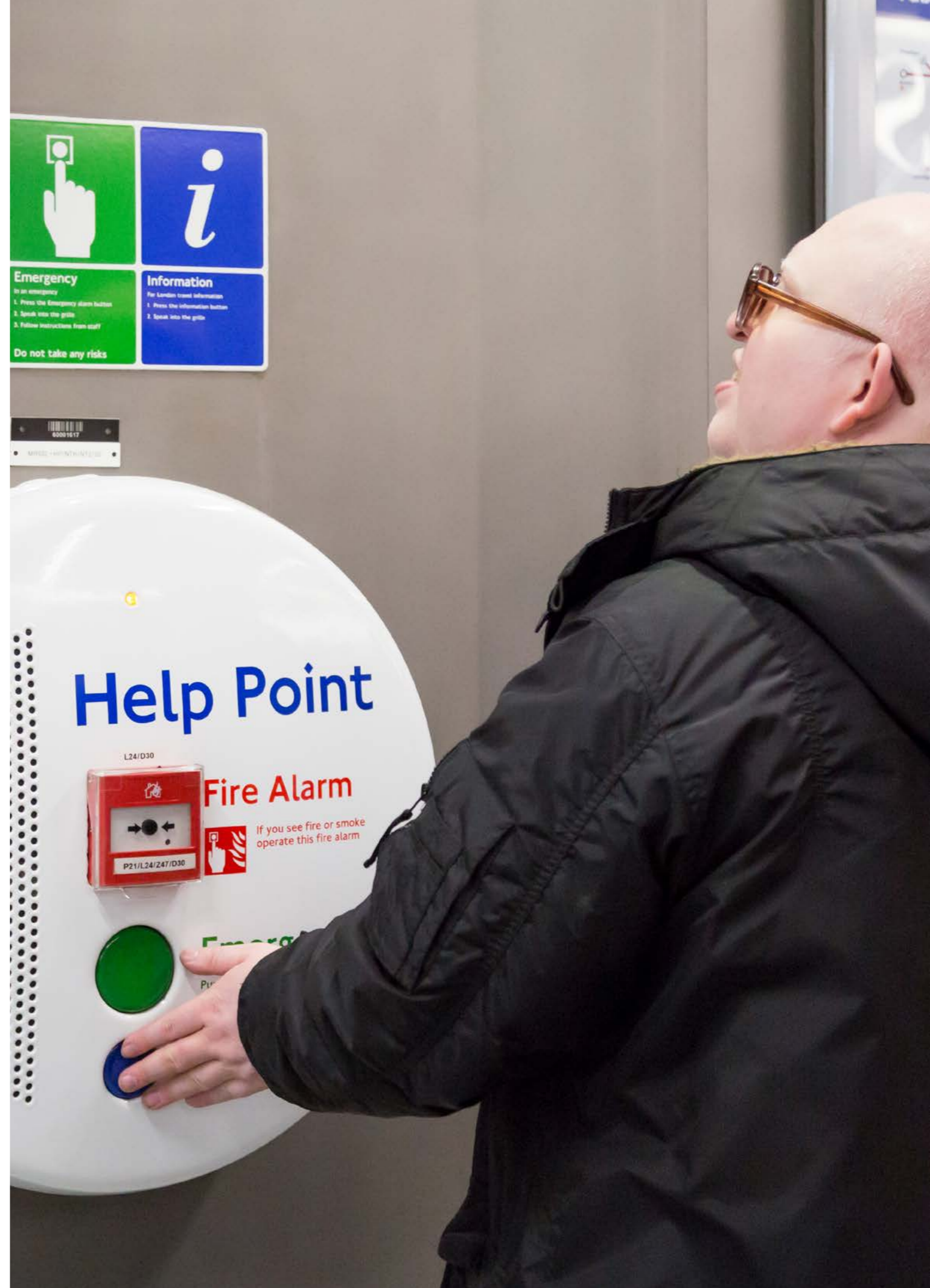
We're improving our station information systems on the Jubilee line
