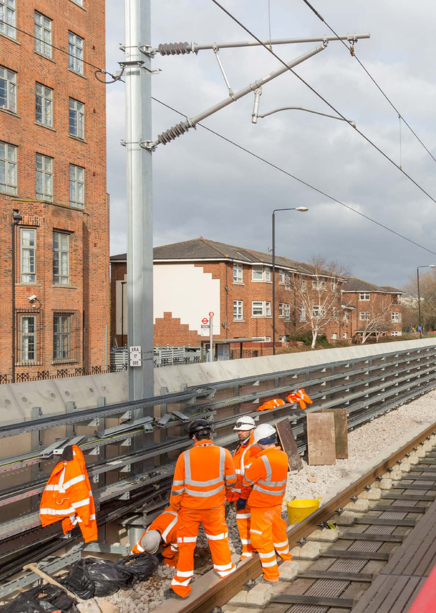
We have converted old rail to a more modern type of track
