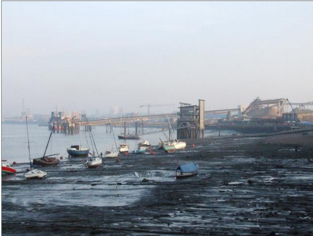
Figure 25: GYC Moorings in foreground at low water and GYC on Pear Tree Wharf in mid shot. Angersteins and Murphy's Wharves to rear (Source: Chris Whippet via: geograph.org.uk ).
