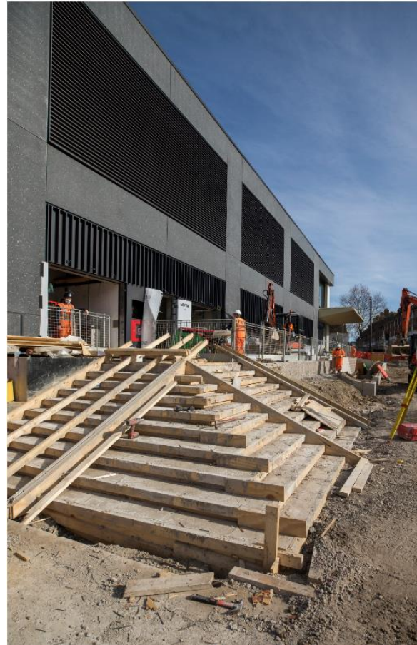
External landscaping under construction
