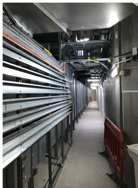
Fig.2 Installation of cabling trays within the shaft
