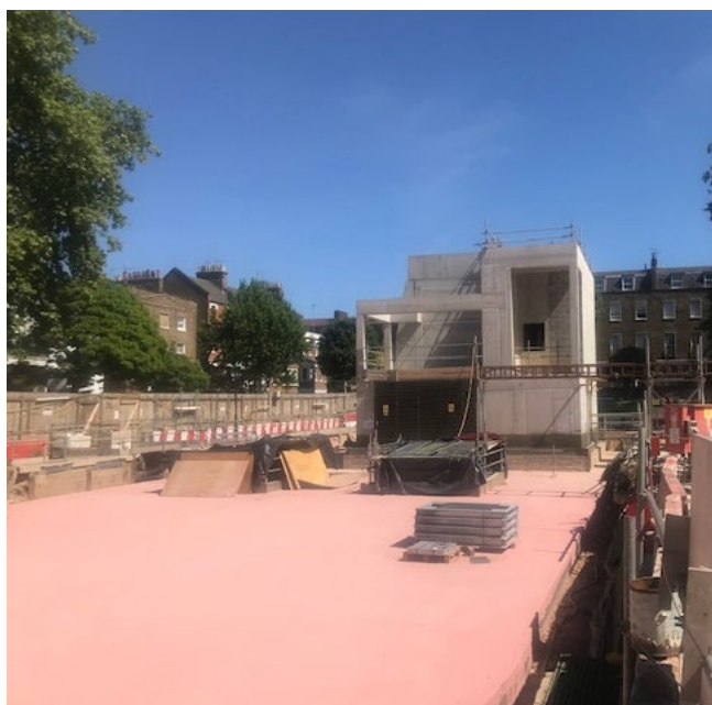
Fig. 1 Waterproofing the basement structure
