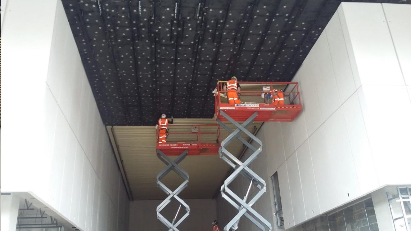
Progress on the ceiling works
