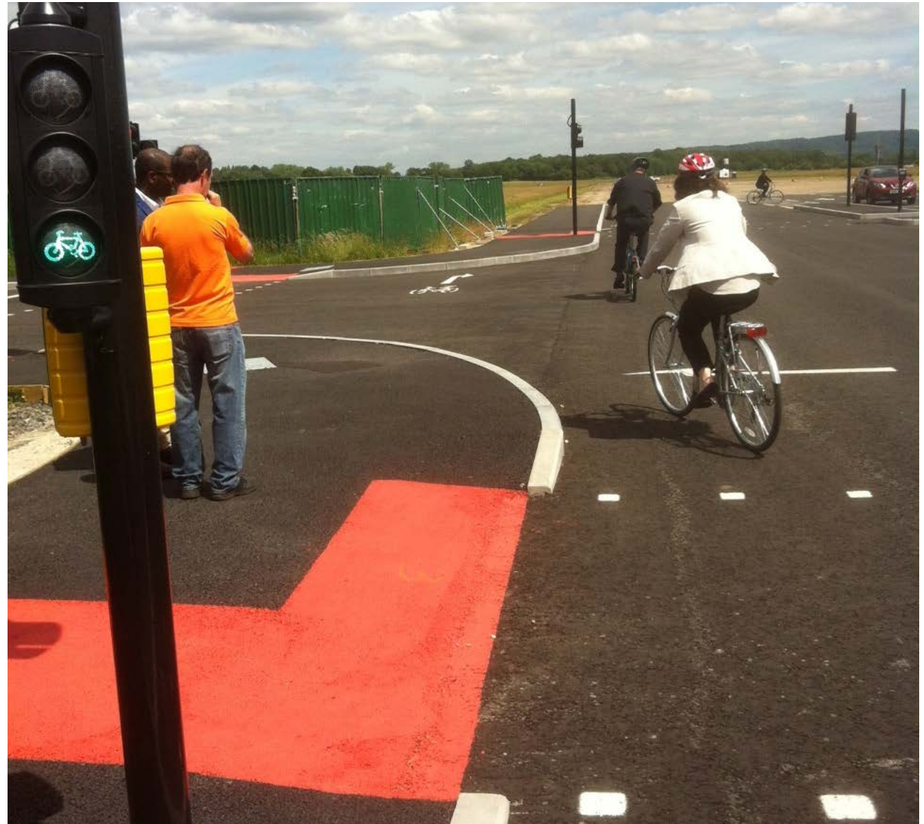
Trial of two-stage right turn, showing low-level cycle signals for early release
