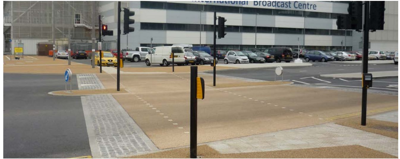
Crossing on a raised table and with contrasting surface treatment, Waterden Road, Hackney
