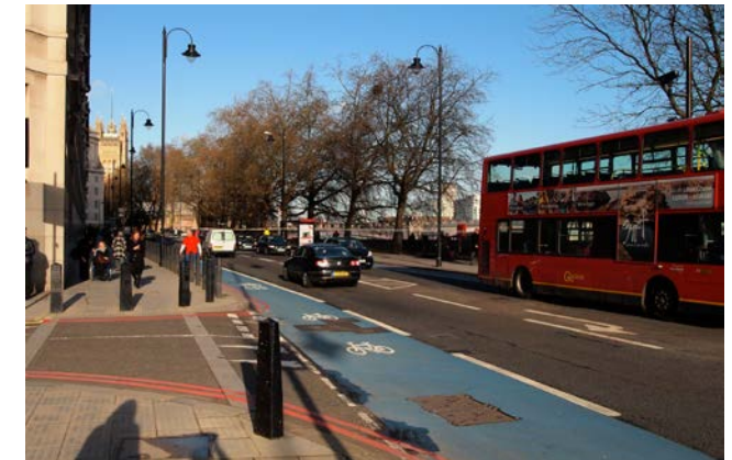
Dashed lane markings continued past side road with raised entry treatment
