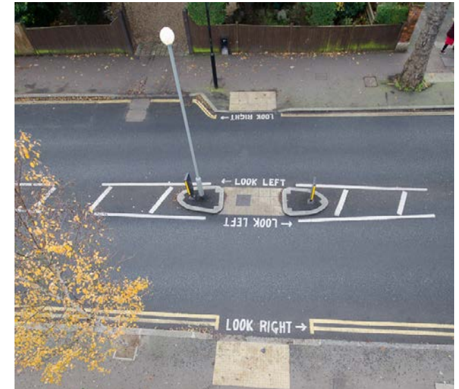
Uncontrolled crossing and refuge islands ('look left' and 'look right' markings not normally needed)
