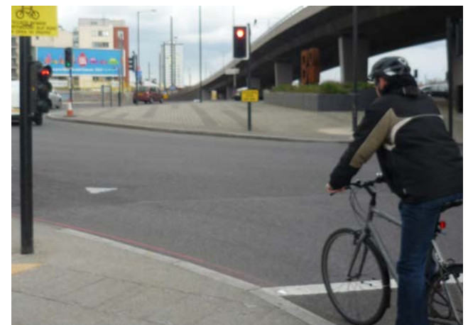
Cycle gate at Bow: (top) segregated approach and first cycle stop line, and (bottom) advanced cycle stop line. Trial low-level cycle signals (used as repeaters) are mounted below the main signal heads
