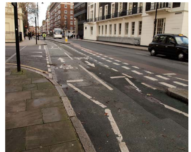
Difficulties in highlighting to all road users that a two-way cycle track is crossing a side road – Tavistock Place, Camden
