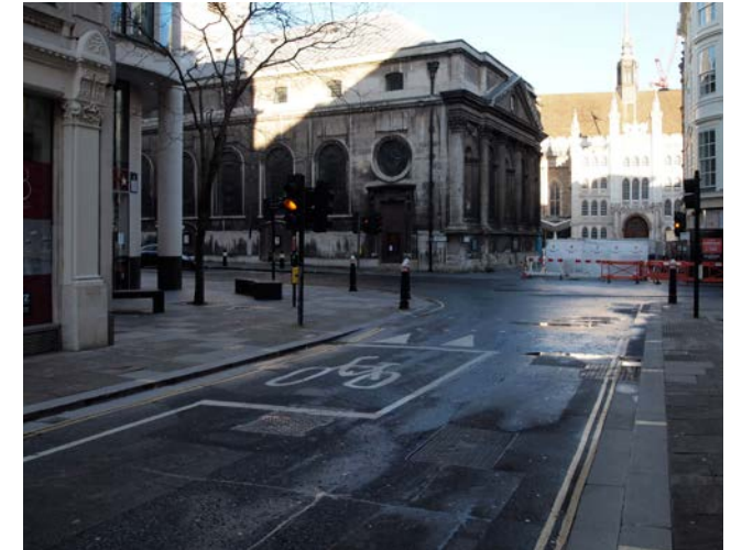
Narrow lead-in lane on street with no centre line, so vehicles tend not to queue over the lead-in lane
