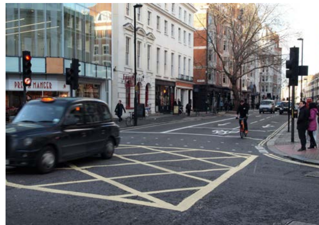
ASL across two lanes only from one-way street (offside lane is a bus lane) – Gower Street, Camden
