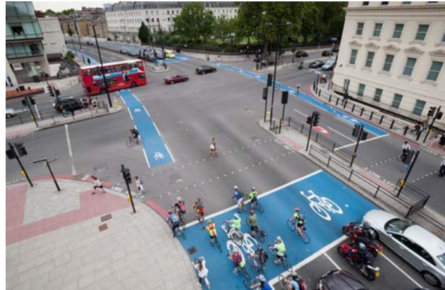
Lane markings and surface colour continued through junctions on Cycle Superhighways
