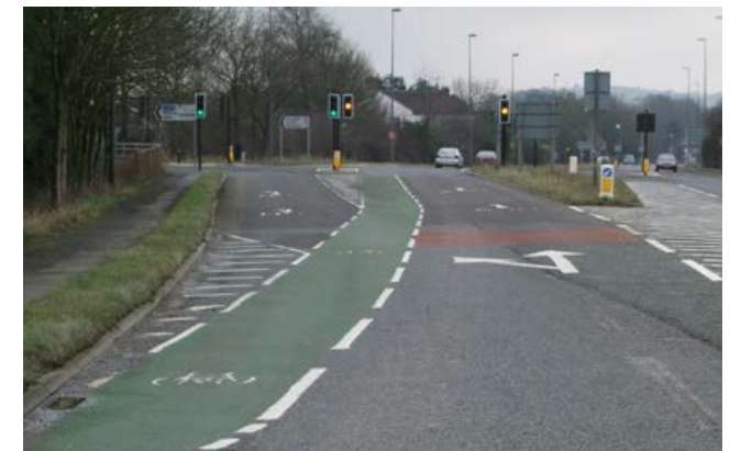
Use of dashed lane markings and surface colour to highlight a cycle lane to motorists seeking to enter a left-turn lane
