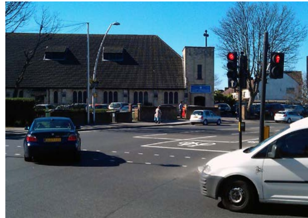
Part-width ASL used where right-turning vehicles would over-run a full-width ASL – Ruckholt Road, Waltham Forest
