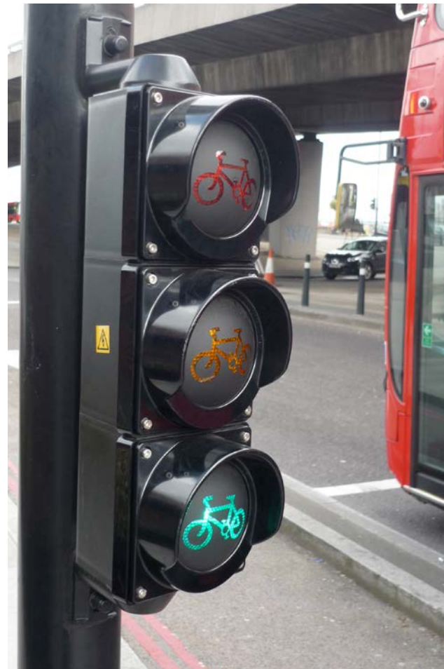
Detail of low-level cycle signal
