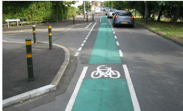
Buffer between lane and give way markings, and use of colour
