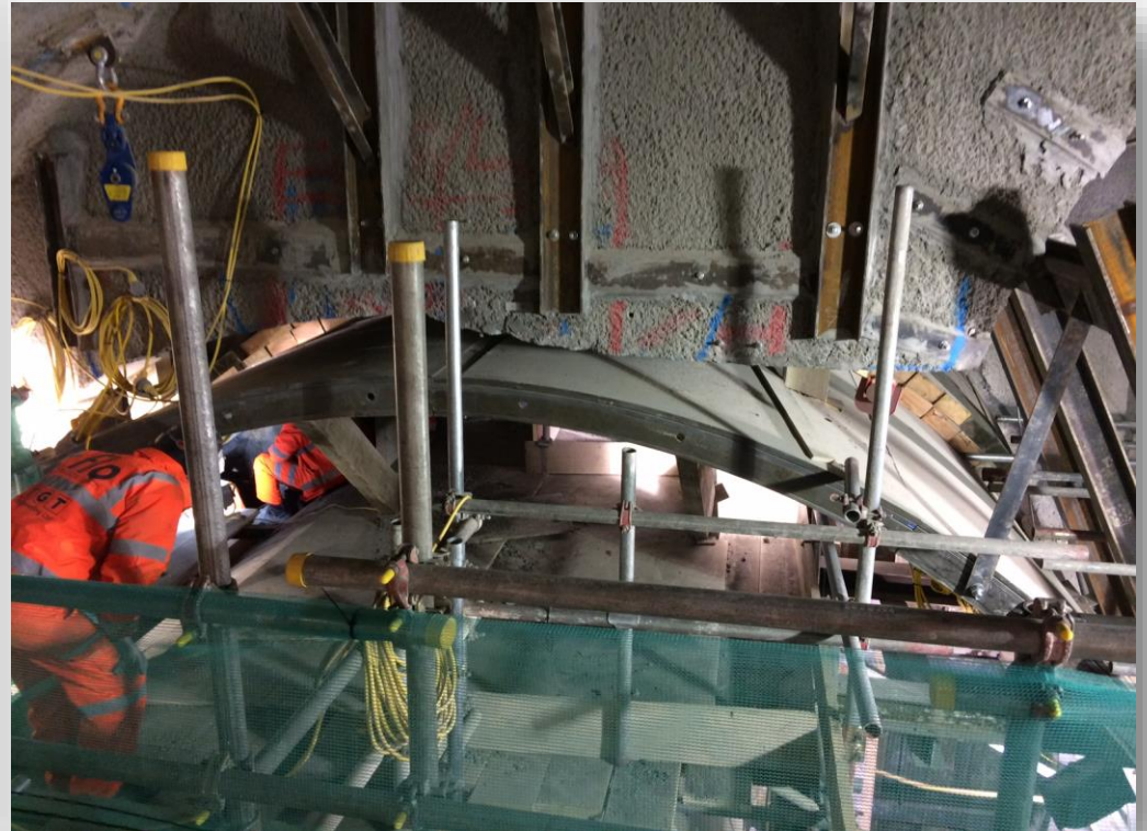
First permanent SGI rings installed W/C – 23/01/2017
