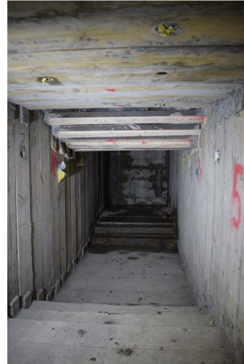
Timber heading excavation WC – 07/11/2016
