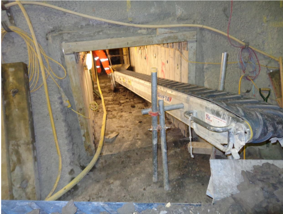
Timber heading excavation WC – 07/11/2016
