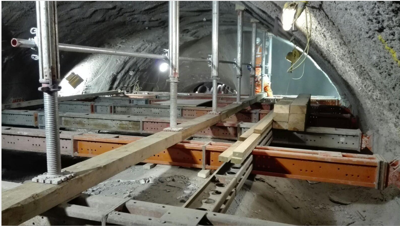
Installation of propping following excavation WC – 17/10/2016
