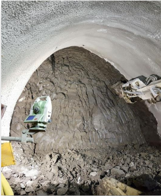
*SCL Pilot tunnel excavation. W/C – 03/10/2016
