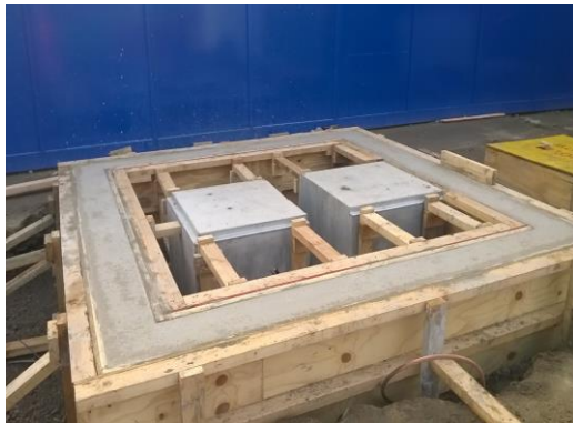
4) Installation of Substation bases
