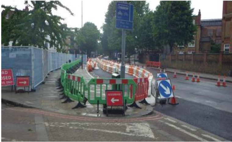
1) Pedestrian footpath reopened
