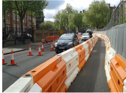
2) Traffic Management in place
