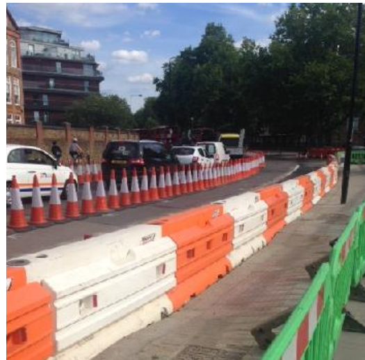
3) Multi utilities reinstated
