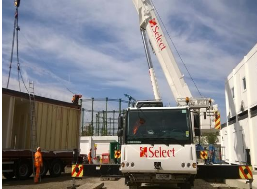
1) Cabin install at Montford Place
