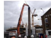
Demolition of the chimney
