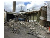
Demolition of the boiler house
