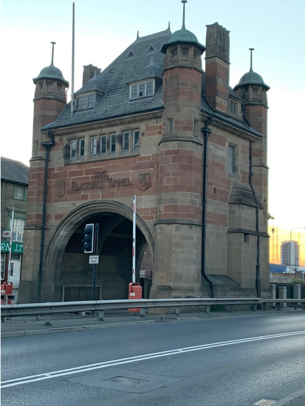
Building 1, South Façade - Photo Taken May 19th 2020
