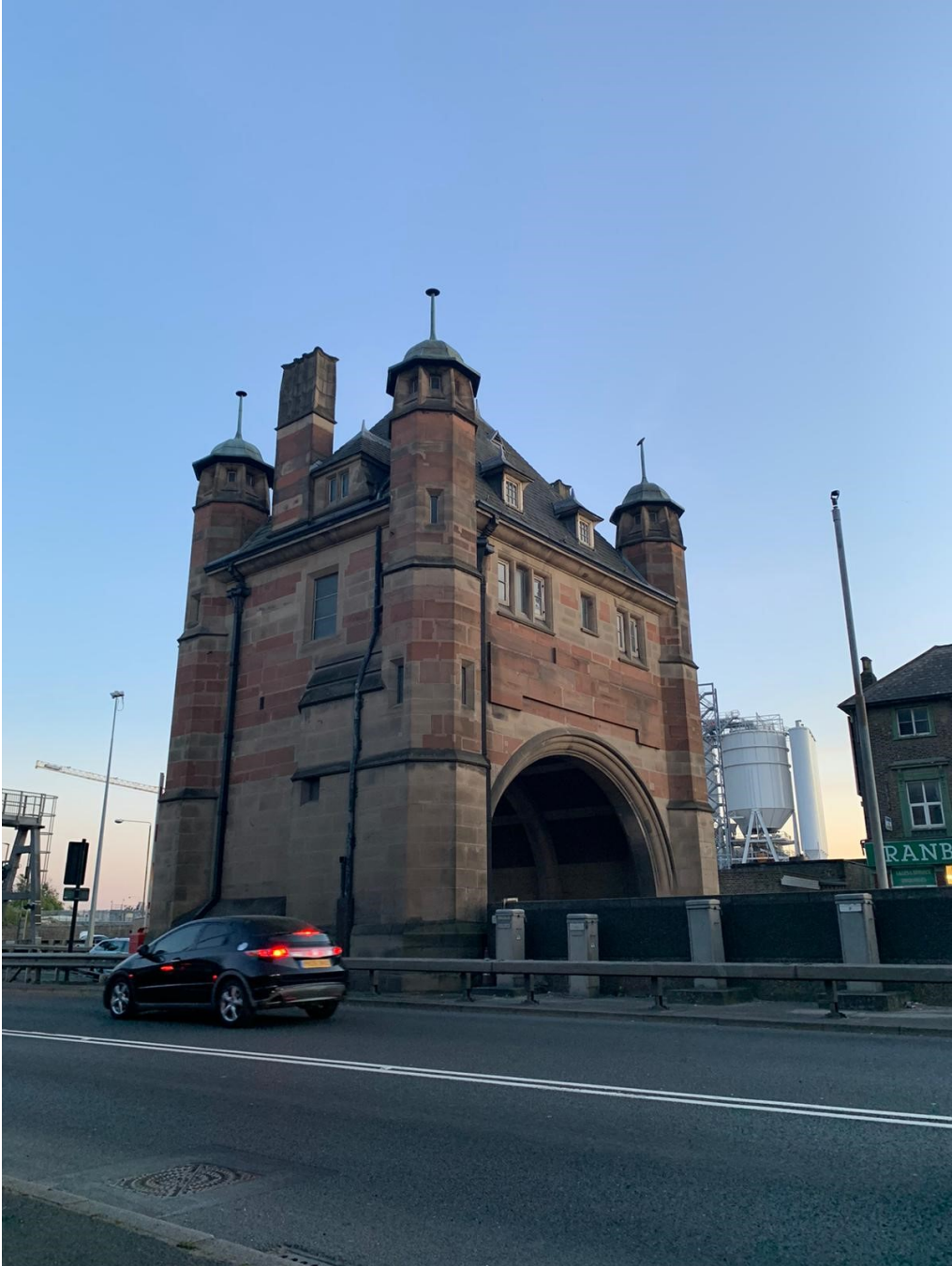
Building 1, North Façade - Photo Taken May 19th 2020
