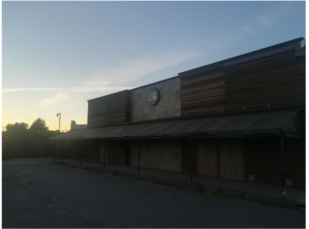
Building 2, West Façade - Photo Taken May 20th 2020
