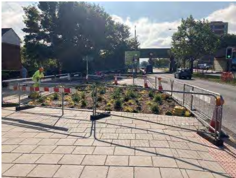
Figure 59. Rain Gardens on TLRN Under Construction in Tolworth (Source: TfL, 2023)
