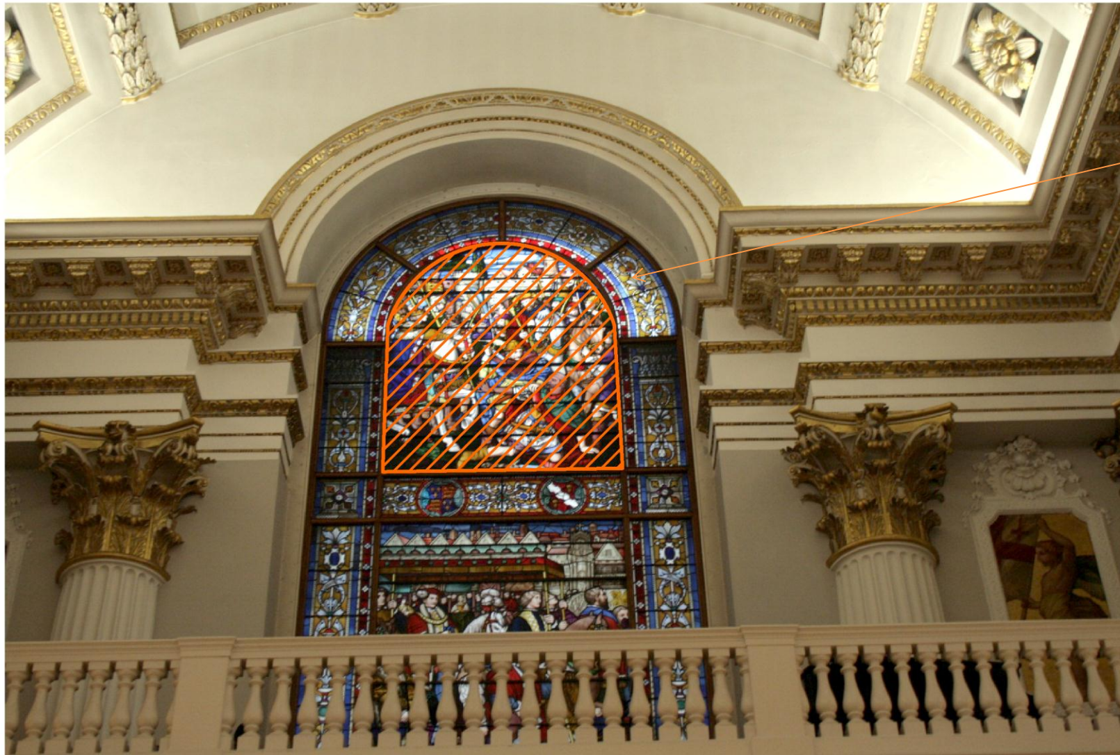
Egyptian Hall eastern window, panel to be temporarily removed
