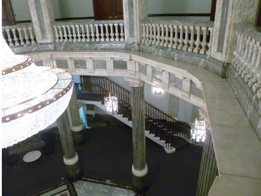
Photo 5: Showing columns and balcony of foyer
