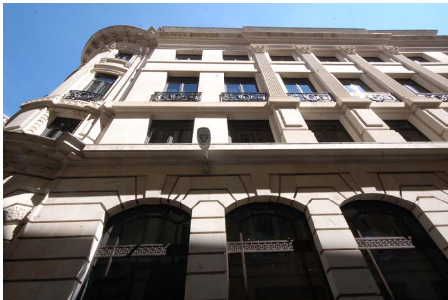
Photo 4: Detail of Sherborne Lane elevation, historic façade with close jointed stone and fine architectural detailing
