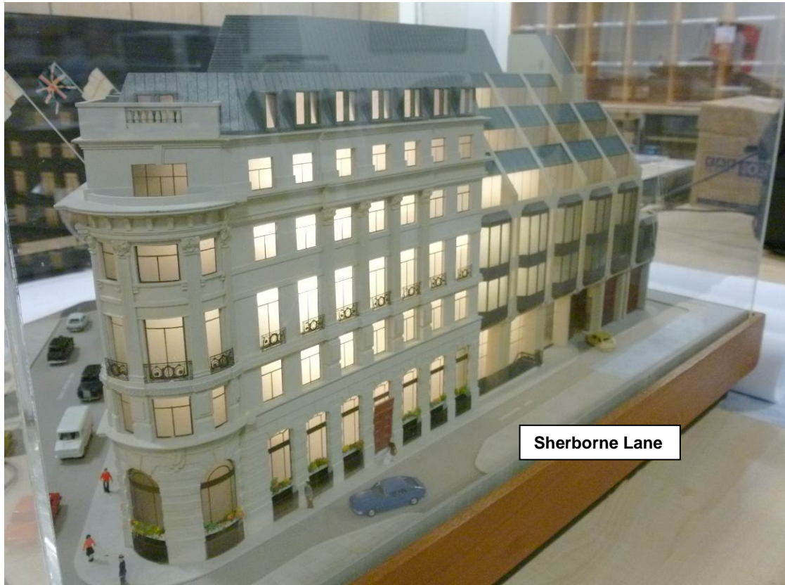
Photo 1: Building model showing Sherborne Lane elevation (retained façade and modern addition), predicted to be subject to the greatest ground movement
