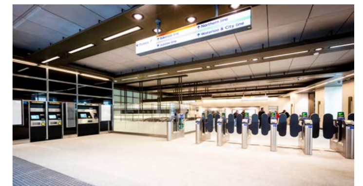
The refurbished York Road entrance to Waterloo
