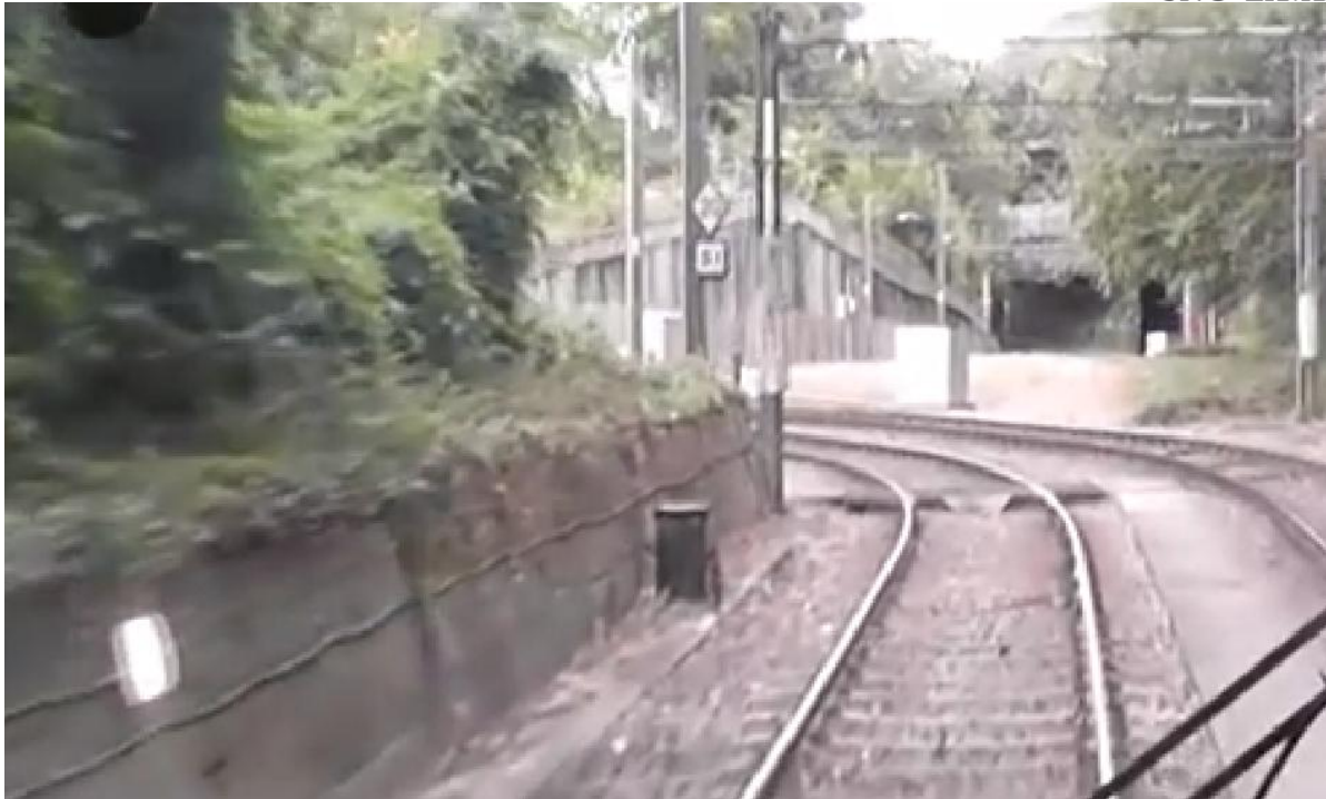
Figure 7 - 20 km/h PSR board on 30m radius curve, with the entrance to the Elmers End/Beckenham Junction branch line showing opposite
