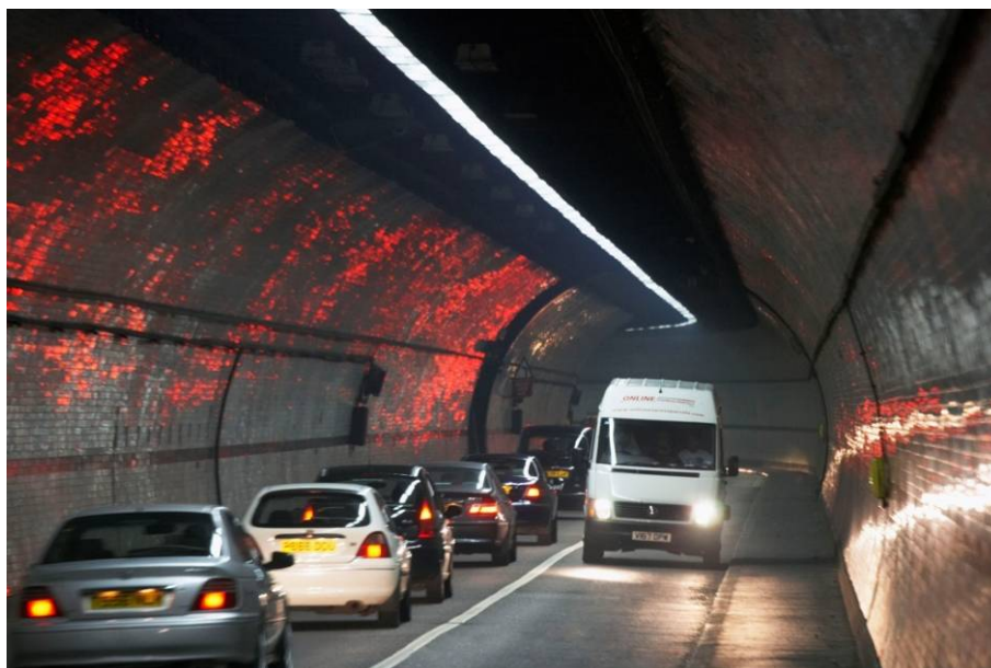
Figure 8.9: Inside the Rotherhithe Tunnel, showing a bend and the narrow footway
