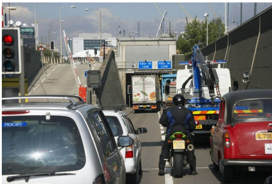
Figure 8.13: Northbound tunnel entry control
