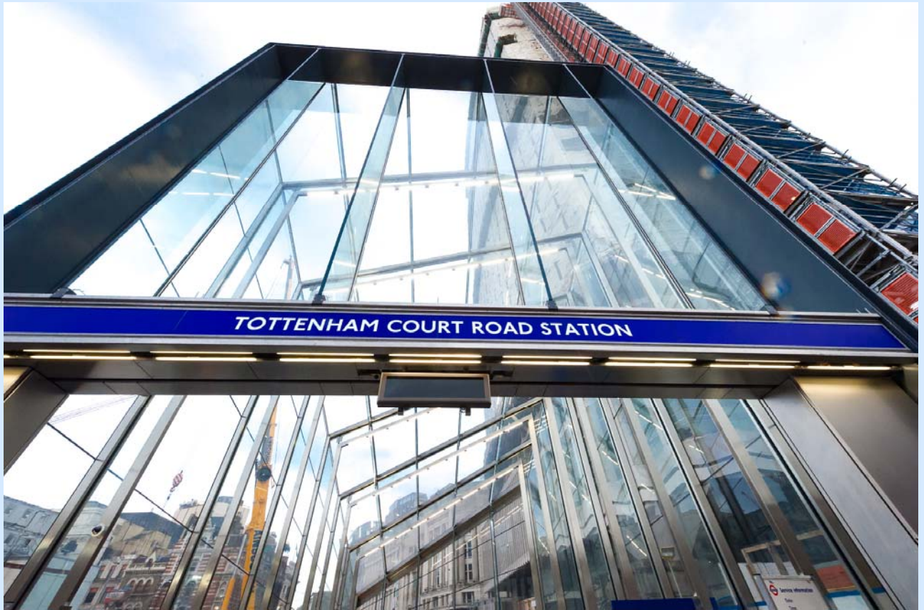
The new south plaza entrance
