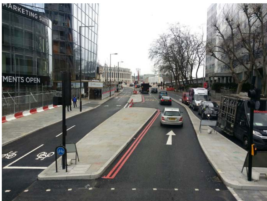
Blackfriars Road following resurfacing
