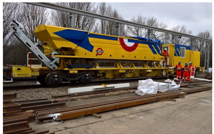
Concrete mixer mounted on donor wagon
