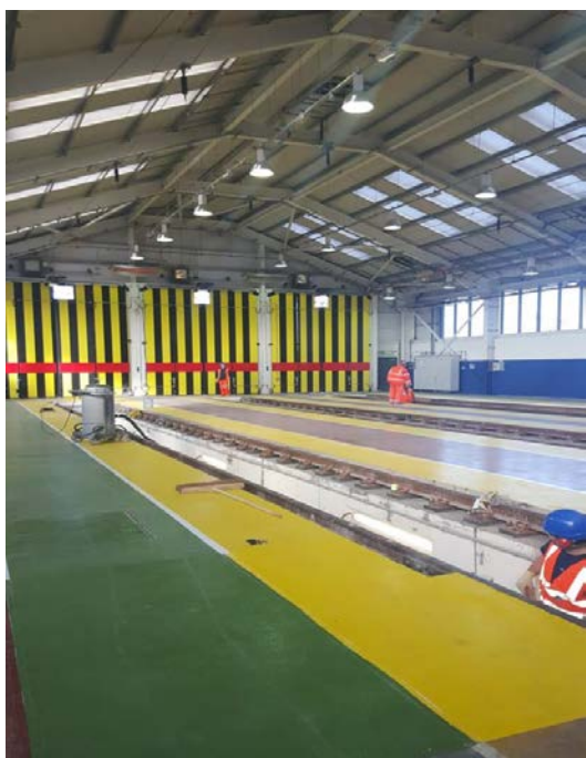
Work is nearing completion at Willesden train depot
