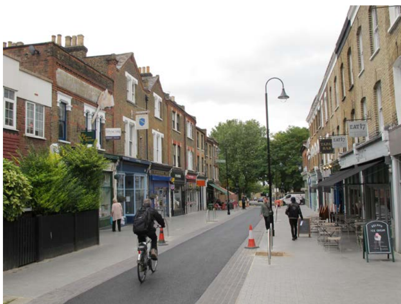
Completed scheme at Pembroke Road/Orford Road in the London Borough of Waltham Forest
