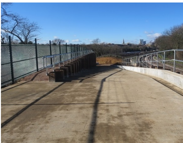
Hanger Lane RRAP Phase I works completed
