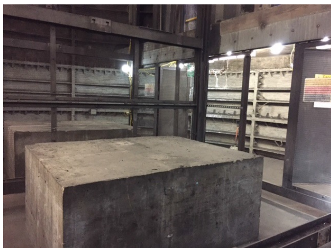
The bottom of the lift shaft at Holland Park
