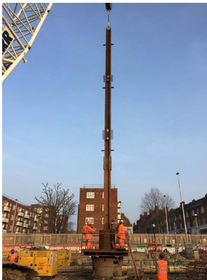
Installation of the first plunge column at Nine Elms site
