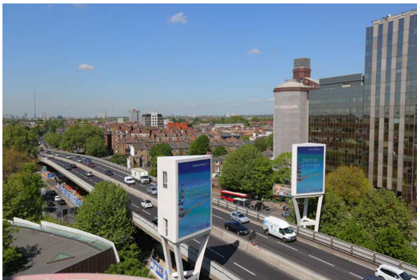
The Hammersmith Flyover
