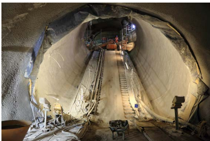
The new escalator shaft
