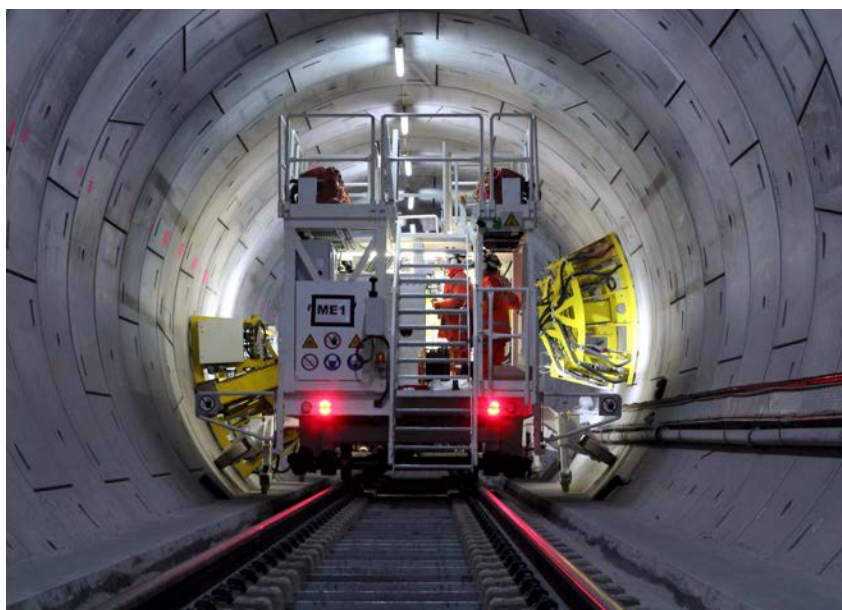
Crossrail's innovative automated drilling machine
