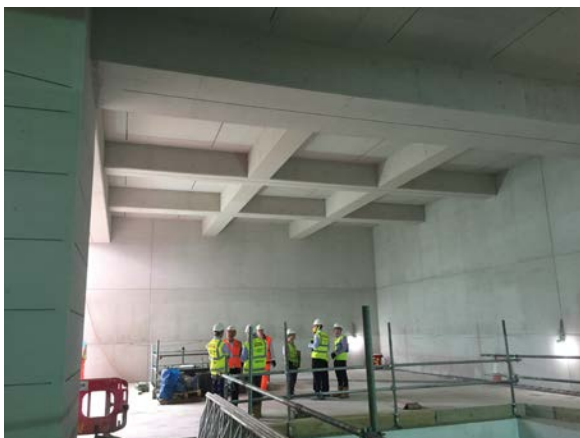
Station box – mezzanine level
