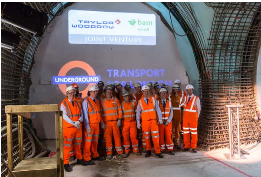
Tunnel breakthrough at Victoria station
