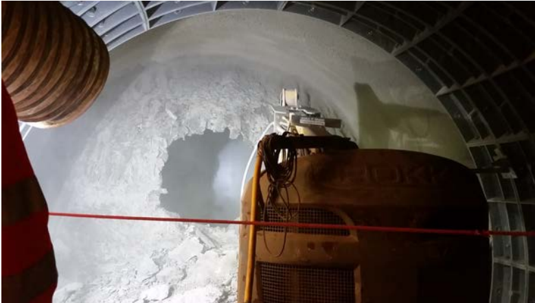
Tunnelling breakthrough at Bond Street station upgrade
