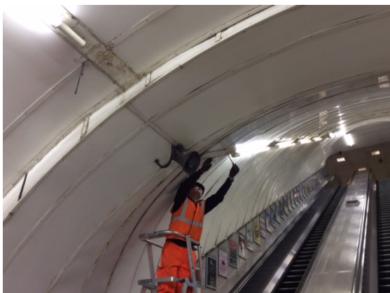
Survey works at Liverpool Street
