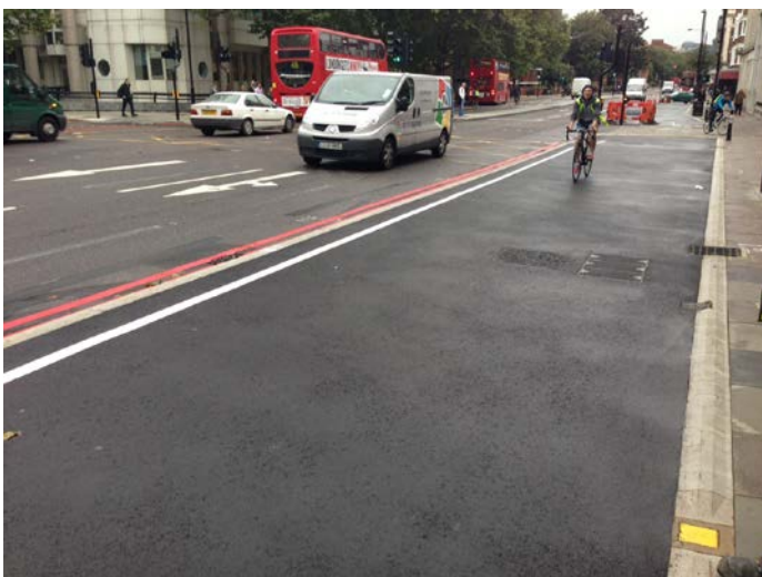
New cycle track on A202 Vauxhall Bridge Road (Cycle Superhighways Route 5 Inner)
