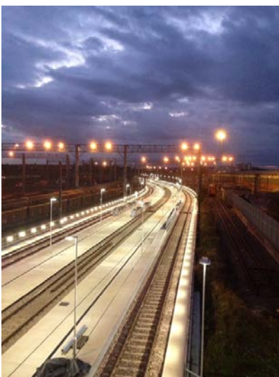
New sidings at Wembley
