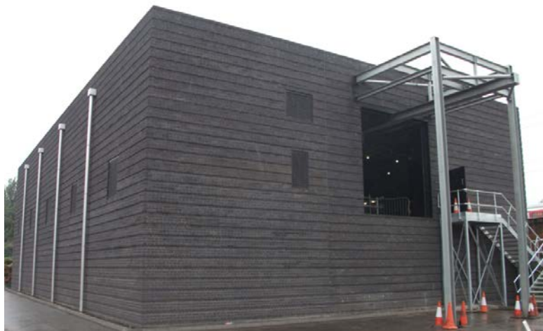
New West Ham high voltage substation
