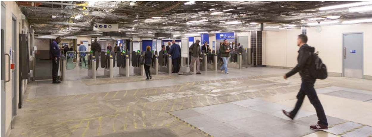
New gateline at Vauxhall station
