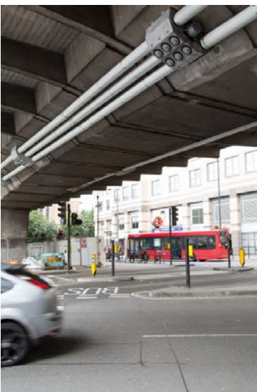
Expansion joint installation at Hammersmith flyover
