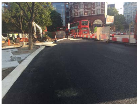
New widened carriageway at London Road junction
