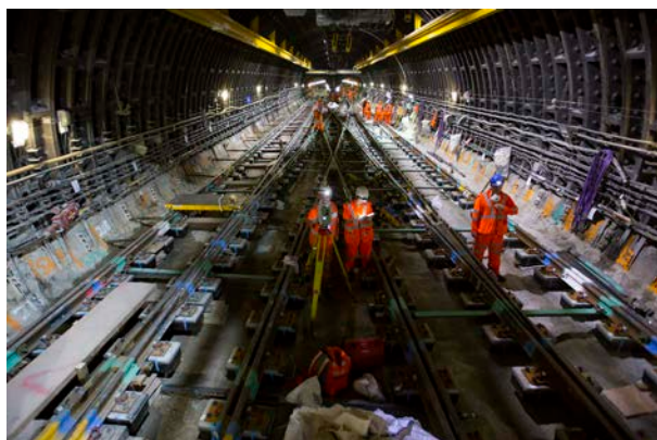
Day 11 of the major renewals at Walthamstow with concrete pouring imminent
