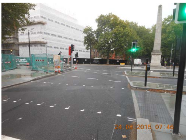
Works in progress at St George's Circus
