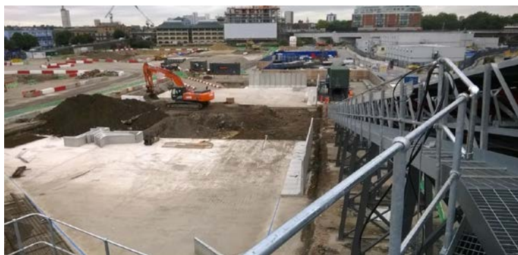
Excavation at Battersea with muck-away conveyor in foreground
