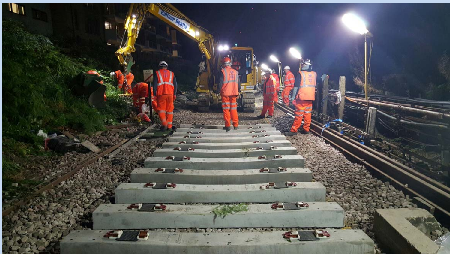
Installation of new ballasted track at White City
