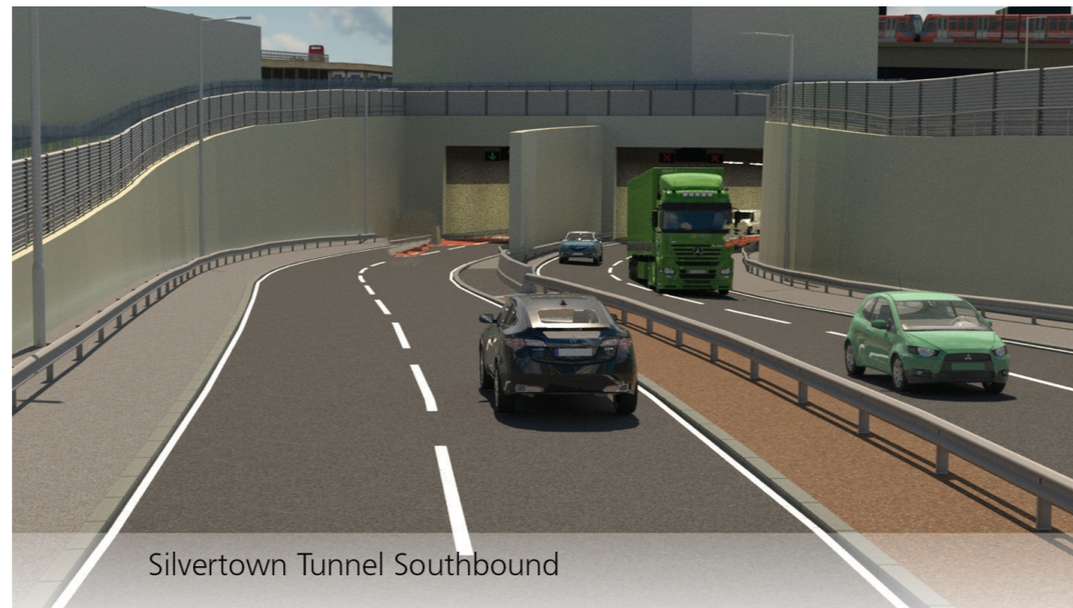
Figure 4.9 – Illustrative view of the Silvertown portal approach ramps and retaining walls from modified Tidal Basin Roundabout looking north
