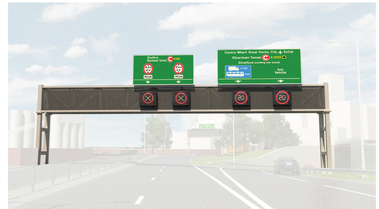
Figure 4.5 – Typical portal truss gantry and VMS signs
