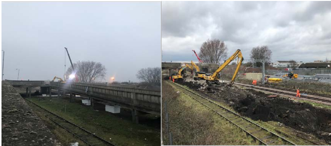
Figure 2: Early Works, Before and After Demolition Works
