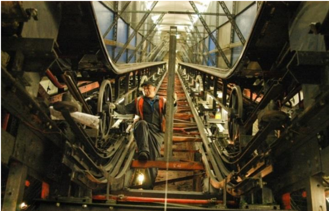
Escalator project works
