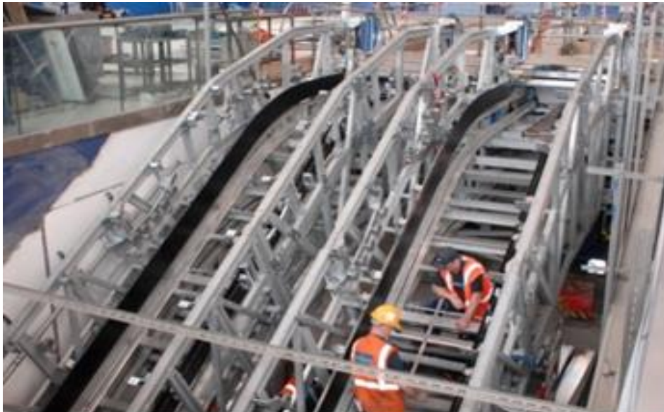
Escalator project works
