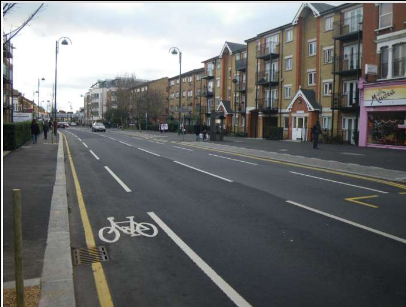
Shared loading space with footway in Leytonstone
