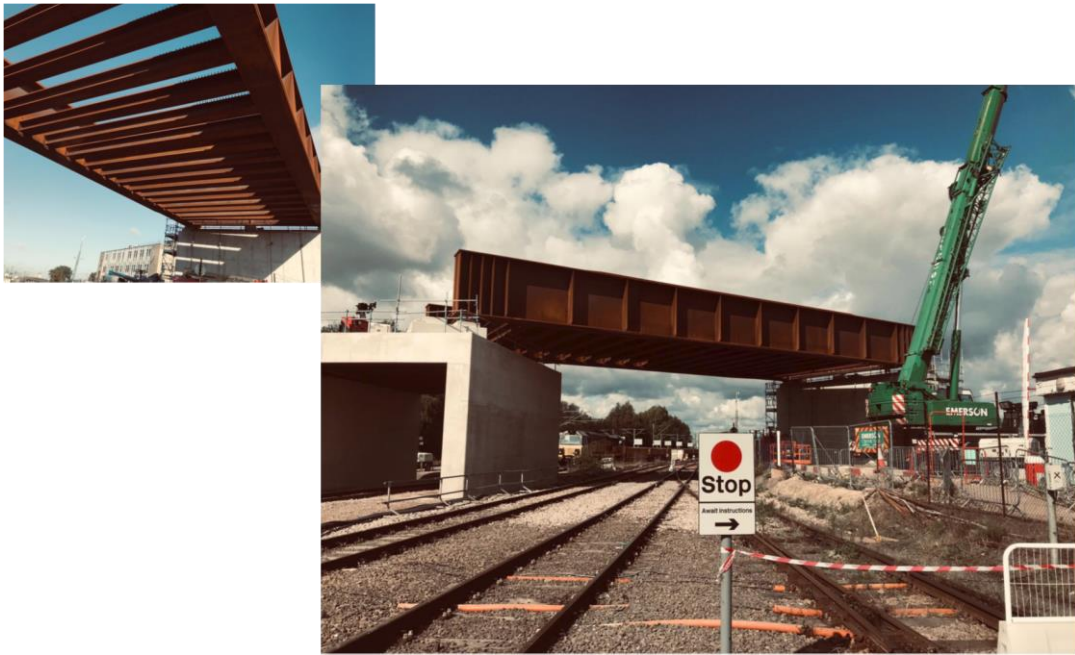
Figure 3: New Span Over Existing Network Rail Infrastructure, August 2020
