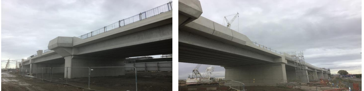
Figure 2: Southern Viaduct nearing completion, October 2020
