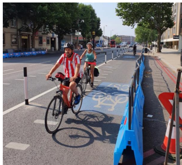
Figure 2: Temporary cycle tracks on Balham High Road which forms part of CS7 between Colliers Wood and Balham.
