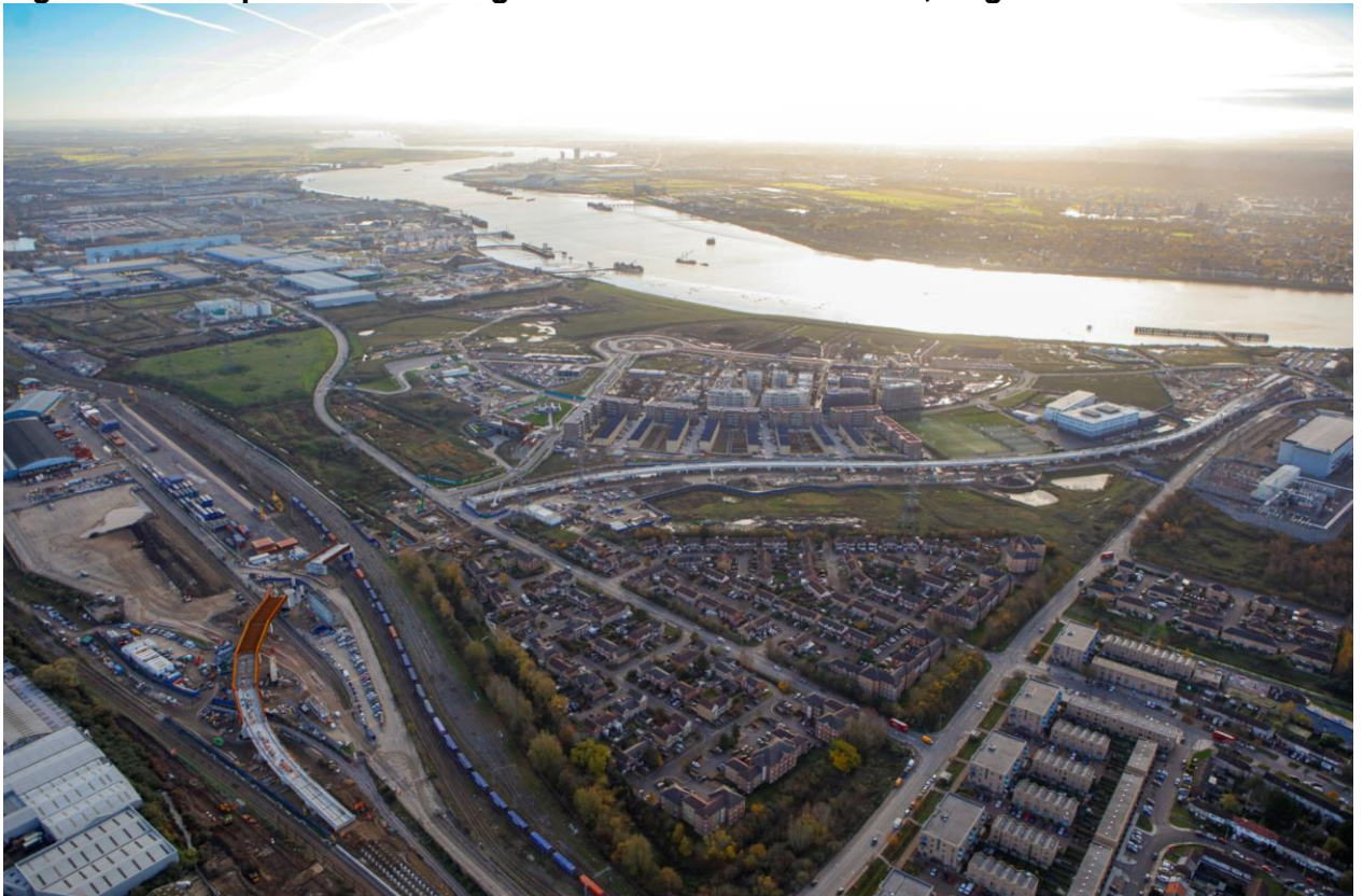
Figure 4: Viaduct Nearing Completion Heading into Barking Riverside, November 2020
