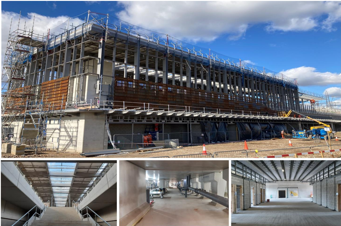
Figure 1: Barking Riverside Station, October 2020
