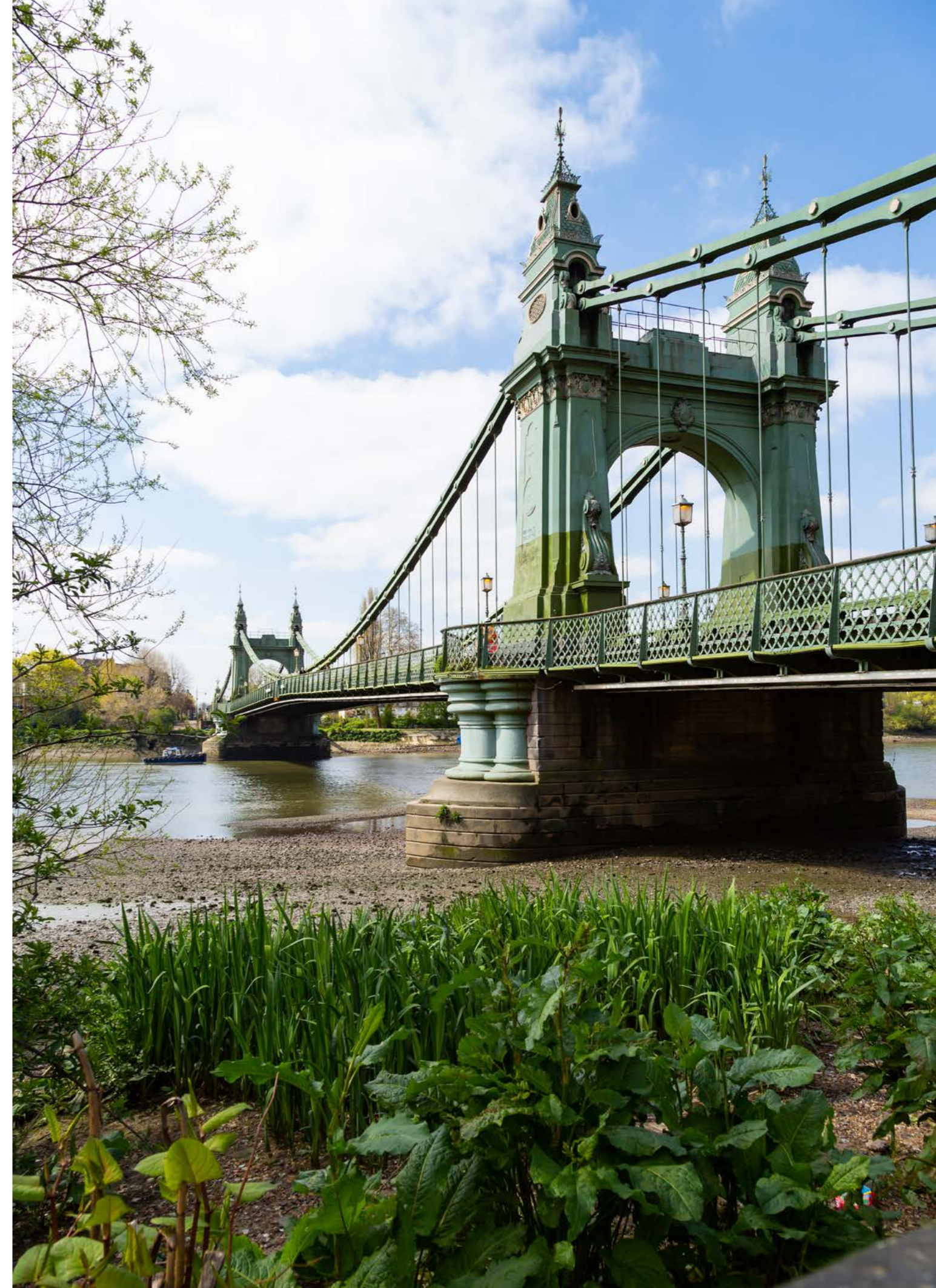
We are contributing to the essential repair work on Hammersmith Bridge
