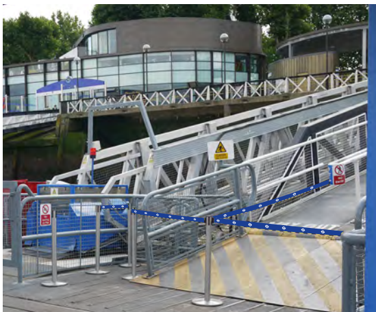
Figure 7. Ramp rider installation for gradients greater than 1/12.
